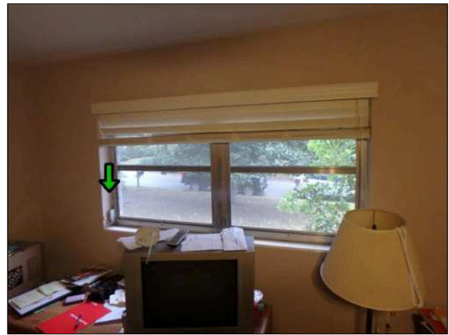
8.3(4) INTERIOR WINDOWS (Picture 10)
