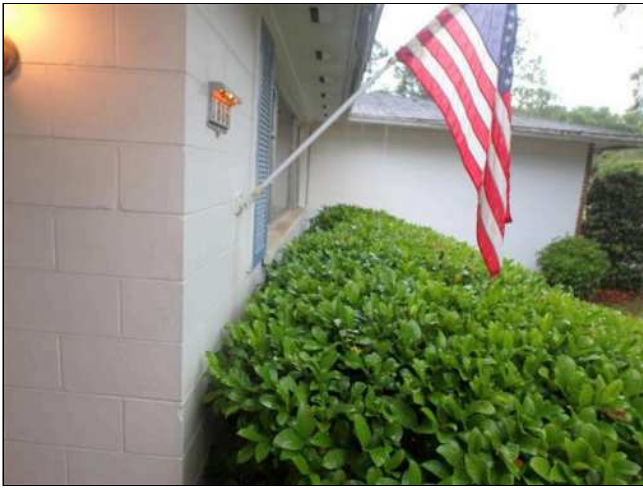
9.0(2) FOUNDATION WALLS (Picture 1)
