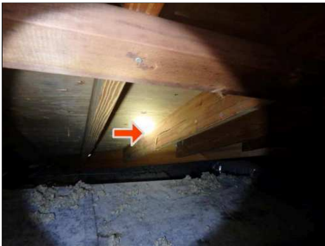
5.0(2) ROOF FRAMING (Picture 1)
