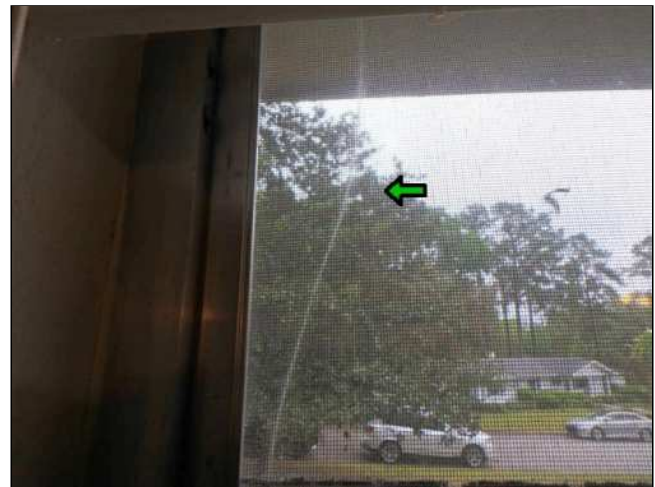
8.3(7) INTERIOR WINDOWS (Picture 4)
