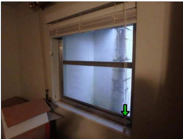
8.3(4) INTERIOR WINDOWS (Picture 1)
