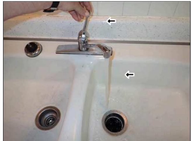
6.0(5) PLUMBING / SINK(S) (Picture 2)
