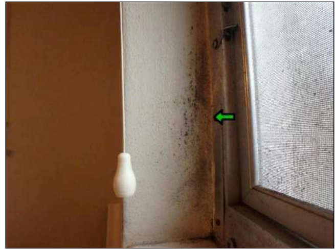
8.3(2) INTERIOR WINDOWS (Picture 2)
