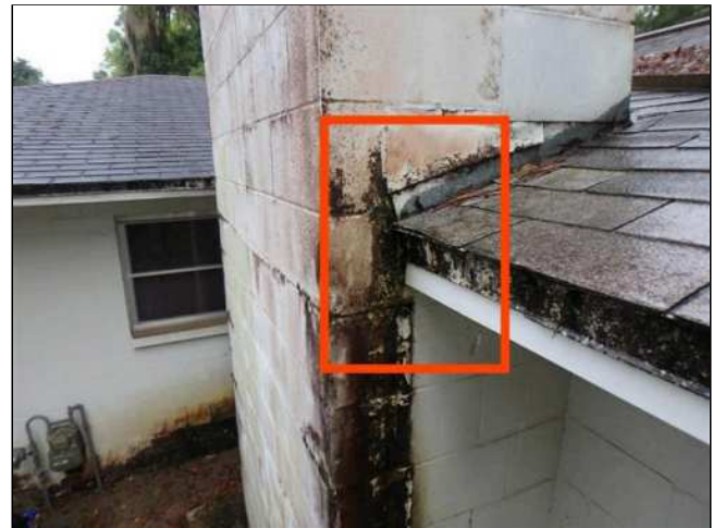
1.2(4) EXPOSED FLASHING (Picture 3)
