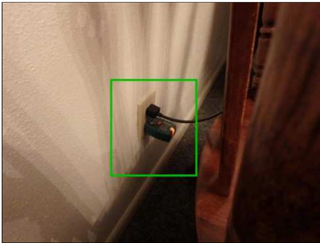
8.7(3) ELECTRIC / DEVICES (Picture 4)
