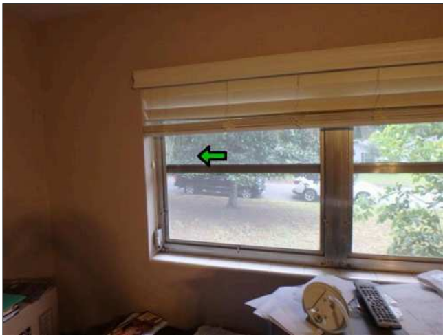
8.3(7) INTERIOR WINDOWS (Picture 3)
