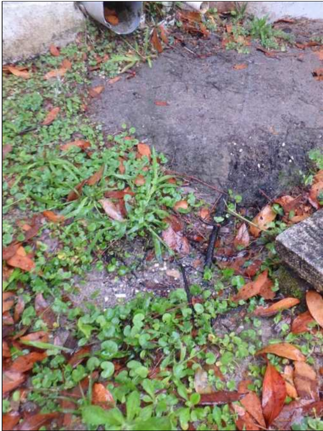
3.4(1) SITE GRADING (Picture 3)
