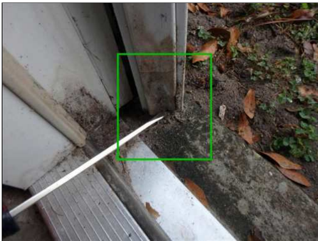
4.9 ENTRY DOOR(S) (Picture 3)
