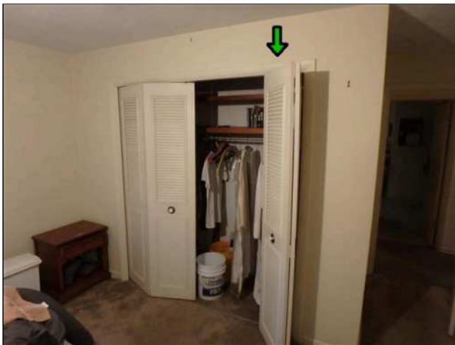
8.5(2) INTERIOR CLOSET DOOR(S) (Picture 3)
