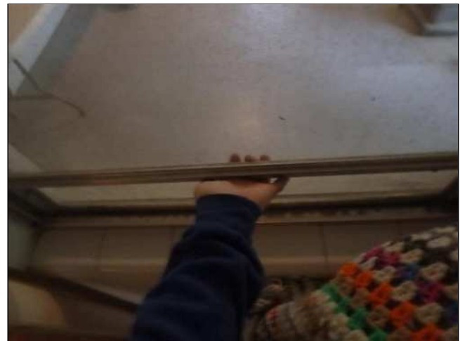
8.3(5) INTERIOR WINDOWS (Picture 3)
