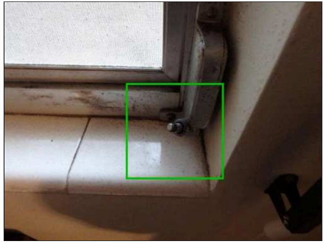
8.3(4) INTERIOR WINDOWS (Picture 4)
