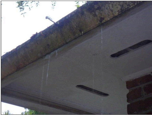
1.7(4) RAIN GUTTERS / EAVESTROUGHES (Picture 2)
