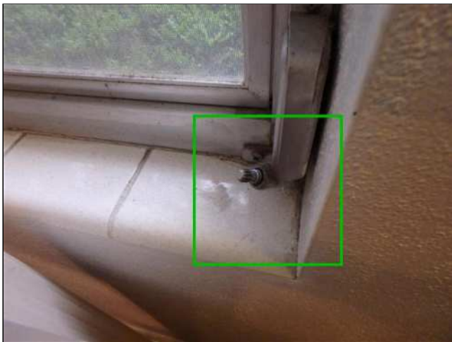
8.3(4) INTERIOR WINDOWS (Picture 7)
