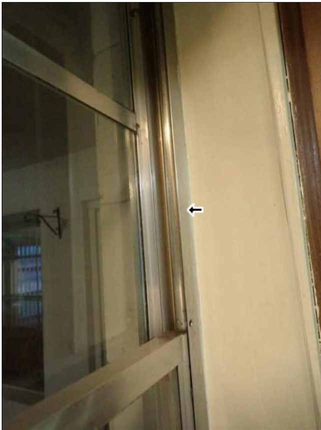
8.3(1) INTERIOR WINDOWS (Picture 3)
