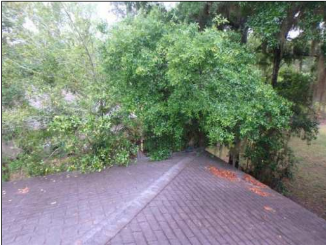
1.0(2) ROOF COVERING (Picture 1)
