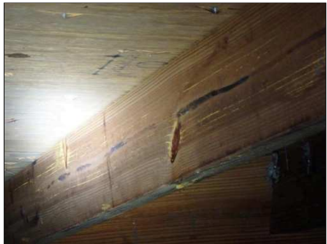
5.0(2) ROOF FRAMING (Picture 2)
