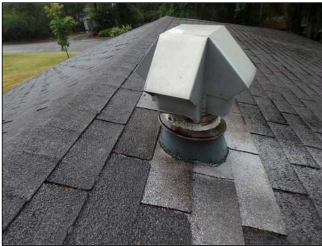
1.2 (3) EXPOSED AND/OR CORRODED HARDWARE OBSERVED AT ROOF FLASHING MATERIALS. Exposed hardware can result in corrosion due to weather conditions which can lead to water intrusion, possibly causing hidden damage. Hardware needs to be sealed in order to maintain roofing / flashing integrity.
