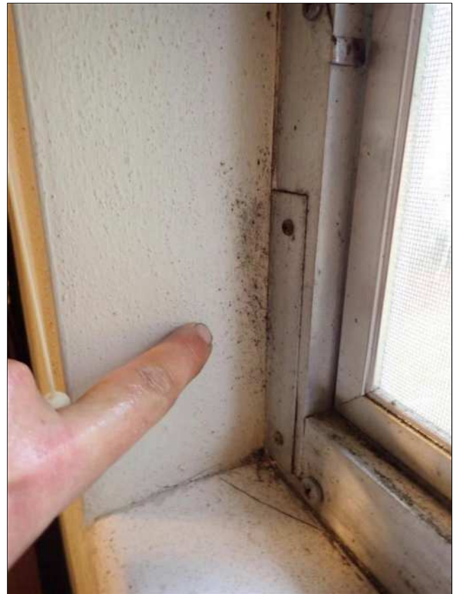
7.27(1) WALLS / CEILING (Picture 6)
