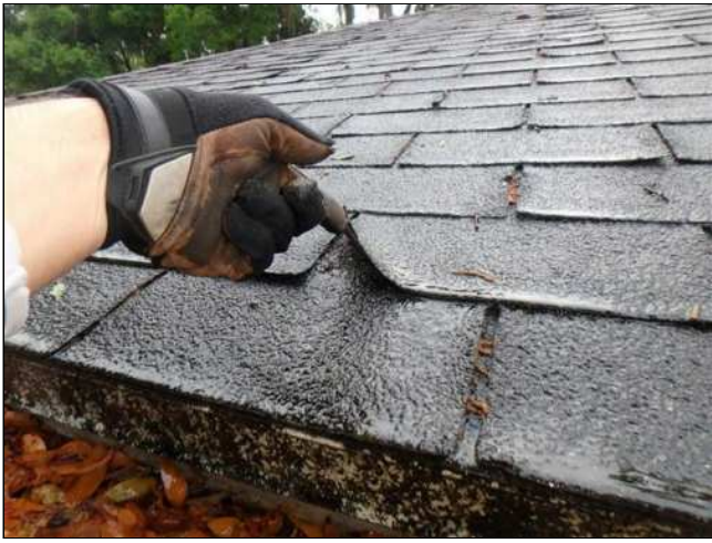
1.0(6) ROOF COVERING (Picture 2)
