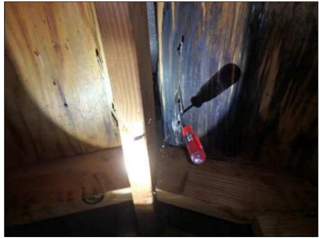
5.1(3) ROOF DECK / SHEATHING (Picture 2)
