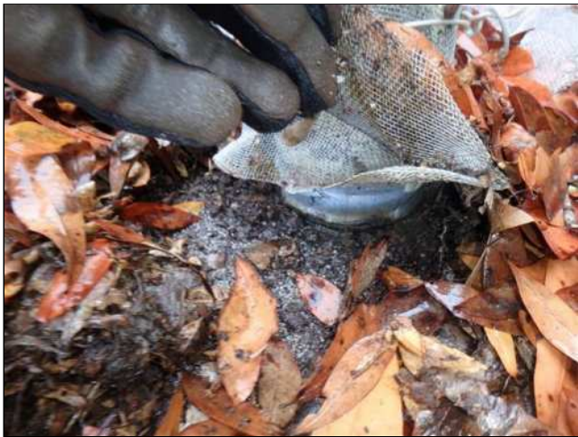
1.2(5) EXPOSED FLASHING (Picture 3)
