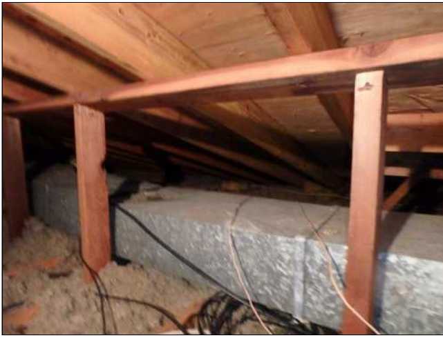
5.0(4) ROOF FRAMING (Picture 1)
