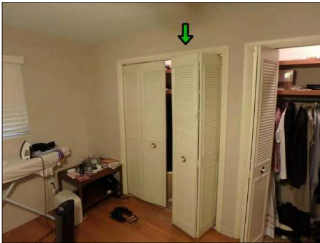
8.5(2) INTERIOR CLOSET DOOR(S) (Picture 1)
