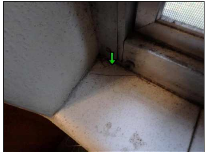
8.3(3) INTERIOR WINDOWS (Picture 2)
