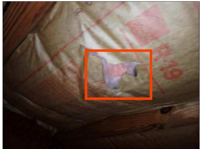
5.4(1) ATTIC ENTRY / ACCESS (Picture 1)
