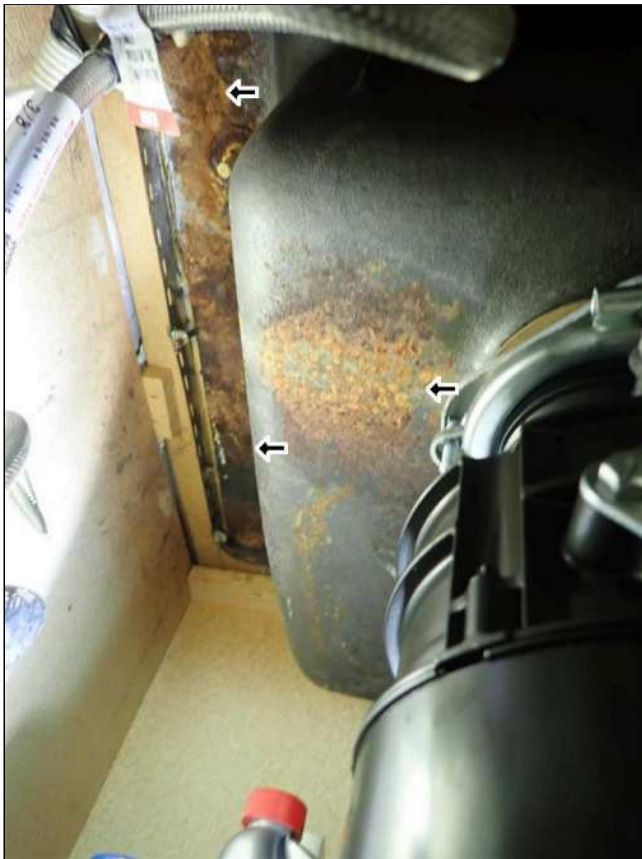
6.0(1) PLUMBING / SINK(S) (Picture 3)
