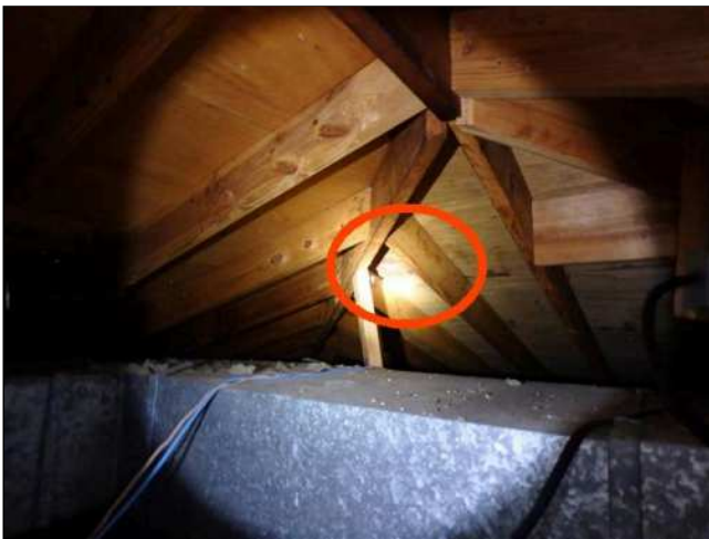
5.1(2) ROOF DECK / SHEATHING (Picture 1)
