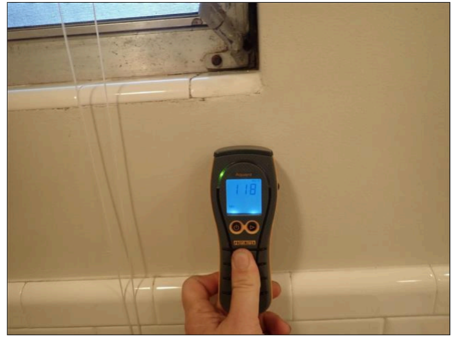
7.18 WALLS / CEILING (Picture 5)
