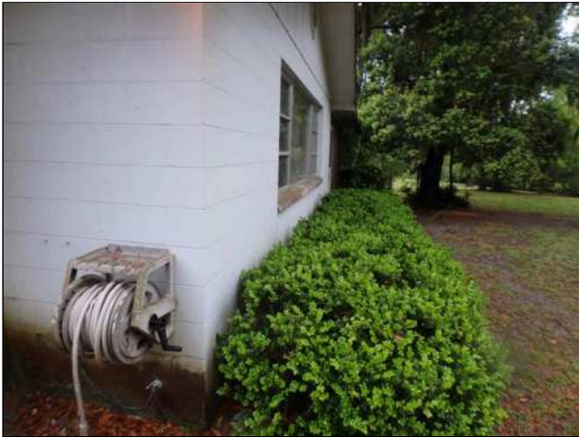
9.0(2) FOUNDATION WALLS (Picture 3)
