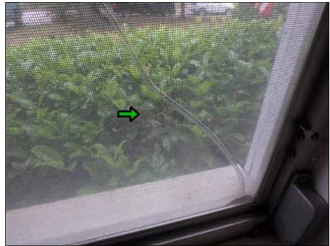
8.3(7) INTERIOR WINDOWS (Picture 2)
