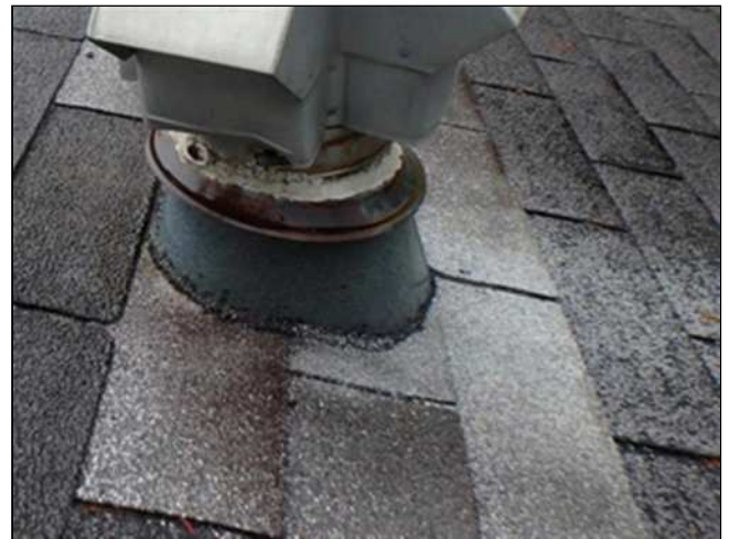
1.2 (3) EXPOSED AND/OR CORRODED HARDWARE OBSERVED AT ROOF FLASHING MATERIALS. Exposed hardware can result in corrosion due to weather conditions which can lead to water intrusion, possibly causing hidden damage. Hardware needs to be sealed in order to maintain roofing / flashing integrity.
