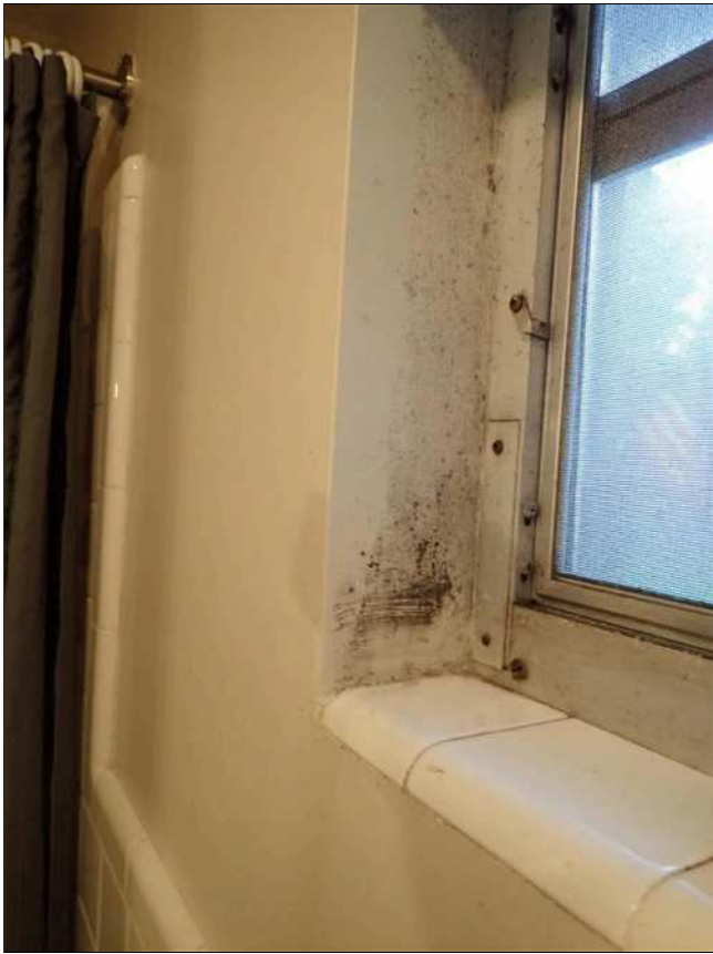
7.18 WALLS / CEILING (Picture 8)
