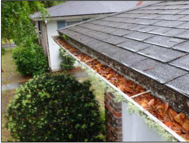
1.7 (2) STAINING OBSERVED AT DOWNSPOUT AND/OR GUTTER SYSTEM SEAMS. THIS IS USUALLY AN INDICATION OF SEAM LEAKS. Full gutters and/or downspout blockage is the primary cause of leaks at the seams of gutters / downspouts. Annual / Bi-annual maintenance may be required in order to ensure gutter / downspout integrity. Pictures shown are a representative number of affected areas.
