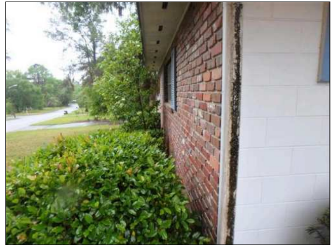
9.0(2) FOUNDATION WALLS (Picture 2)
