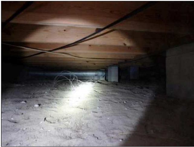
9.6 CRAWLSPACE ENTRY / ACCESS (Picture 2)
