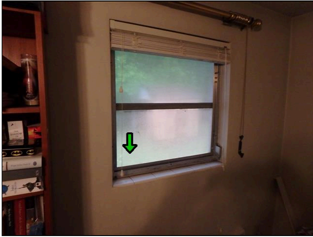
8.3 (4) MISSING CRANKS / HARDWARE OBSERVED AT REAR AND RIGHT SIDE WINDOWS OF RIGHT FRONT BEDROOM, THE REAR FAMILY ROOM WINDOWS AND THE FRONT WINDOWS AT LEFT FRONT BEDROOM. Condition may make window difficult to operate. Windows functioned normally at time of inspection.
