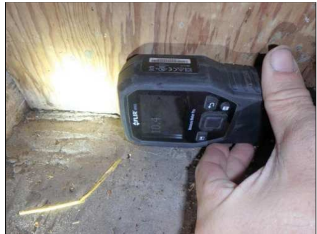
4.4(2) WALLS / CEILINGS (Picture 4)
