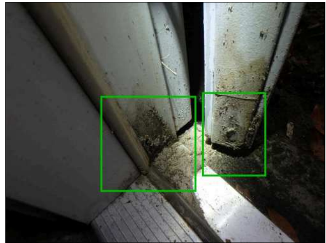
4.9 ENTRY DOOR(S) (Picture 2)
