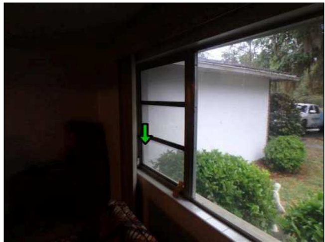
8.3(4) INTERIOR WINDOWS (Picture 8)
