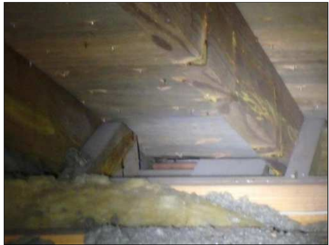
5.0(1) ROOF FRAMING (Picture 6)
