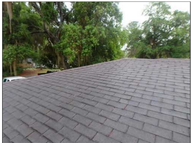
1.0(7) ROOF COVERING (Picture 1)
