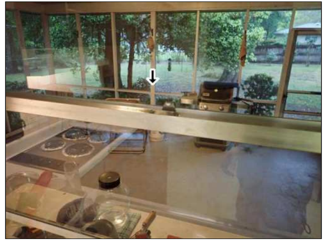
8.3(1) INTERIOR WINDOWS (Picture 2)
