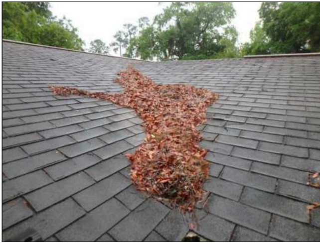
1.0(3) ROOF COVERING (Picture 1)
