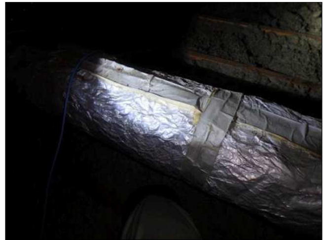
5.7 HVAC SYSTEM PROVISIONS (Picture 1)
