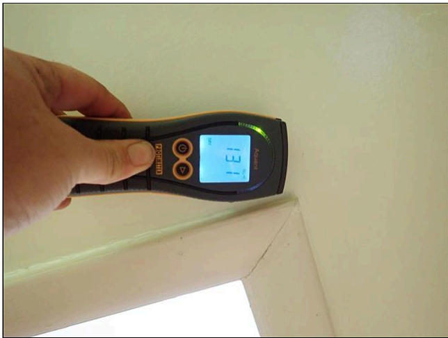
6.2 WALLS / CEILING (Picture 3)
