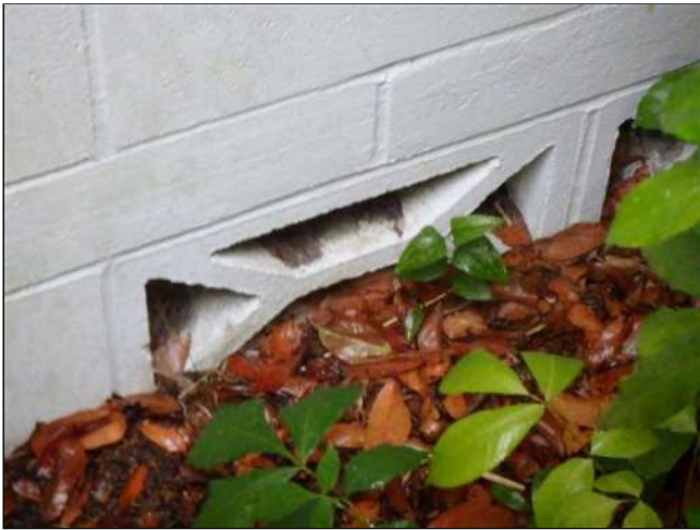
9.5 CRAWLSPACE VENTILATION PROVISIONS (Picture 2)
