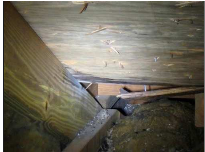
5.0(1) ROOF FRAMING (Picture 2)
