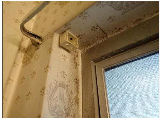
7.27(1) WALLS / CEILING (Picture 2)
