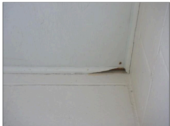
1.8(2) FASCIA / SOFFITS (Picture 2)
