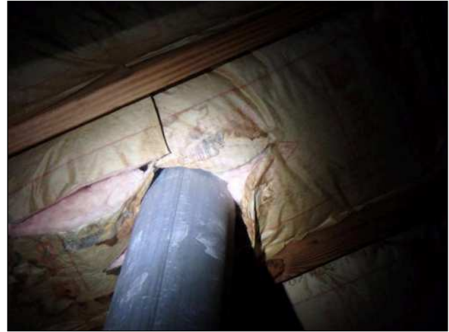
4.4(1) WALLS / CEILINGS (Picture 2)
