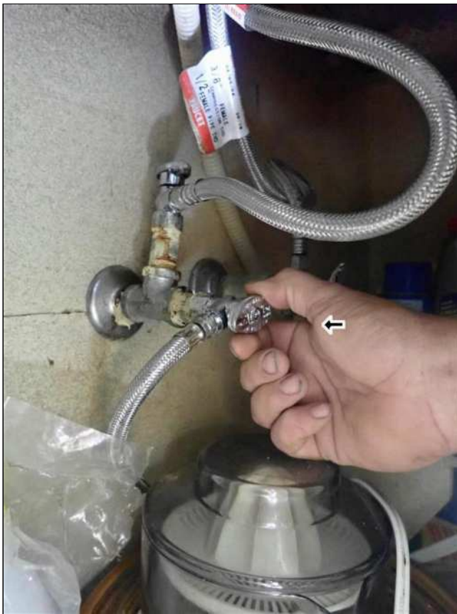
6.0(2) PLUMBING / SINK(S) (Picture 1)
