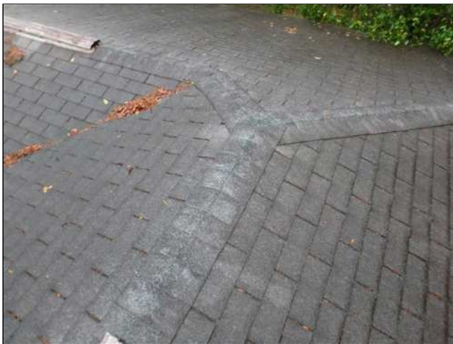
1.0(5) ROOF COVERING (Picture 1)
