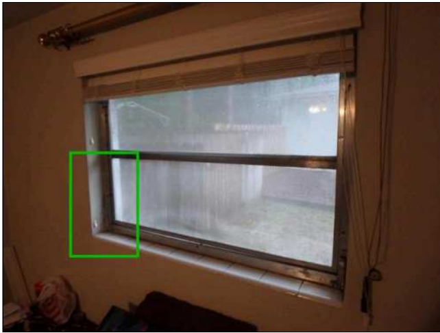
8.3(2) INTERIOR WINDOWS (Picture 1)
