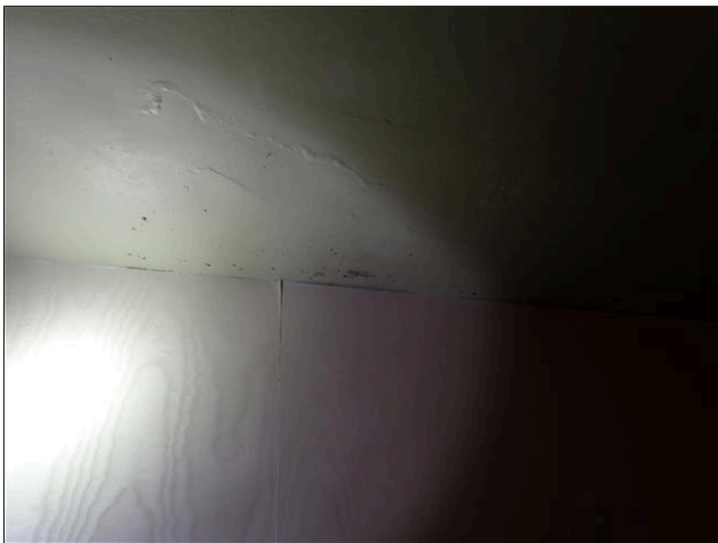
7.7 WALLS / CEILING (Picture 4)
