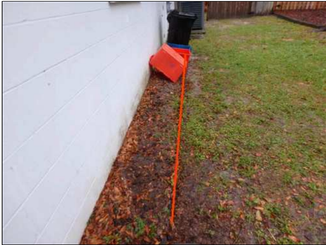
3.4(1) SITE GRADING (Picture 1)
