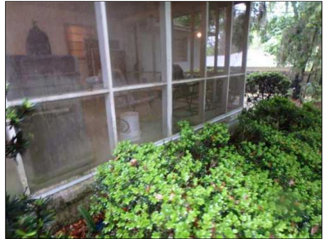
9.0(2) FOUNDATION WALLS (Picture 4)
