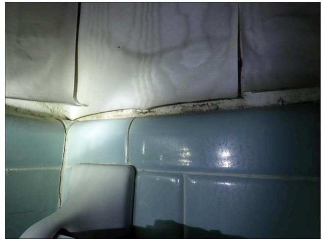
7.7 WALLS / CEILING (Picture 3)
