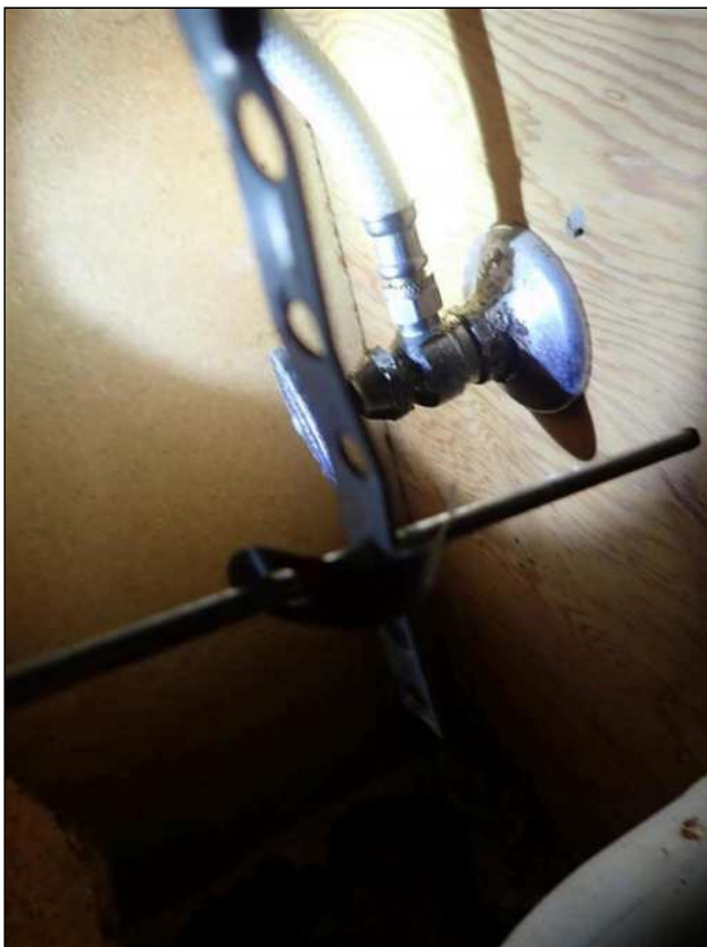
7.1 (2) STOPPER MECHANISM DOES NOT COMPLETELY CLOSE STOPPER TO BE ABLE TO FILL SINK.
