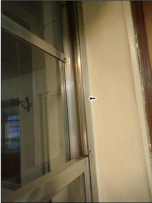
8.3 (2) MICROBIAL GROWTH / MILDEW OBSERVED AT THE RIGHT SIDE WINDOW OF RIGHT FRONT BEDROOM. Condition is normal due to sweating from thermal variation / non-insulated windows.
