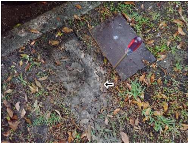
14.7(1) WATER METER (Picture 1)
