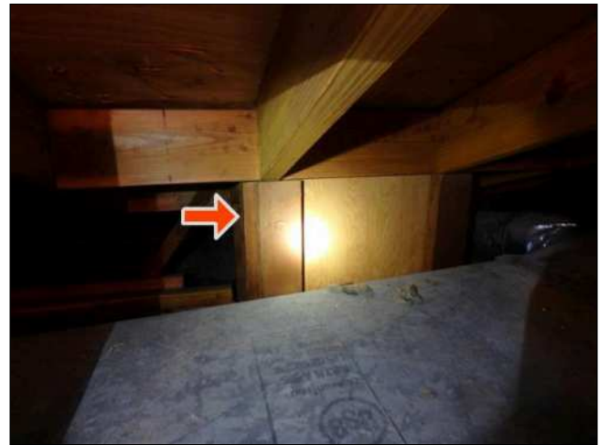
5.6 SKYLIGHT ENCLOSURE (Picture 2)
