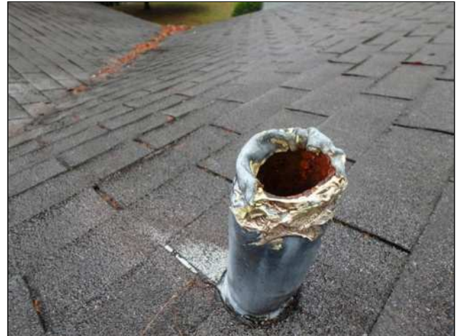
1.2(1) EXPOSED FLASHING (Picture 2)
