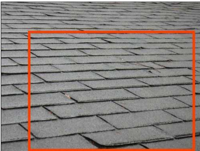
1.0(6) ROOF COVERING (Picture 6)
