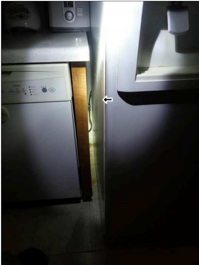
6.0(4) PLUMBING / SINK(S) (Picture 1)
