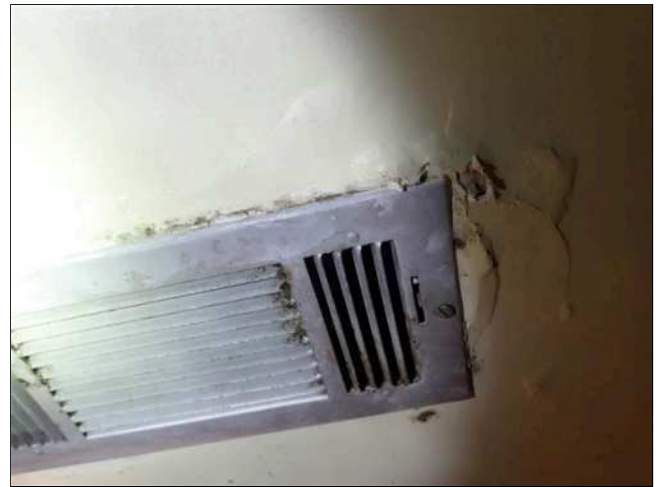
7.7 WALLS / CEILING (Picture 9)
