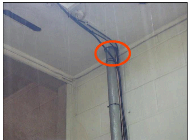
1.8(1) FASCIA / SOFFITS (Picture 1)
