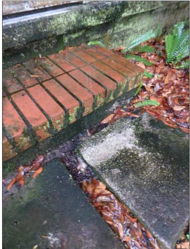
3.4(1) SITE GRADING (Picture 8)
