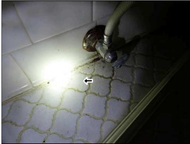
7.13 (4) TOILET SEAT WAS FOUND BROKEN AT TIME OF INSPECTION.
