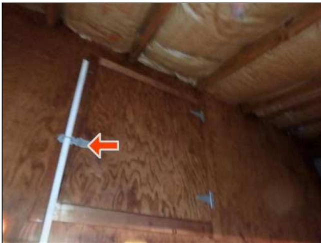
5.4(2) ATTIC ENTRY / ACCESS (Picture 1)
