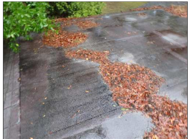
1.1(4) ROOF COVERING 2 (Picture 1)
