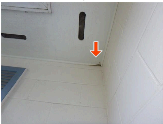
1.8(2) FASCIA / SOFFITS (Picture 1)
