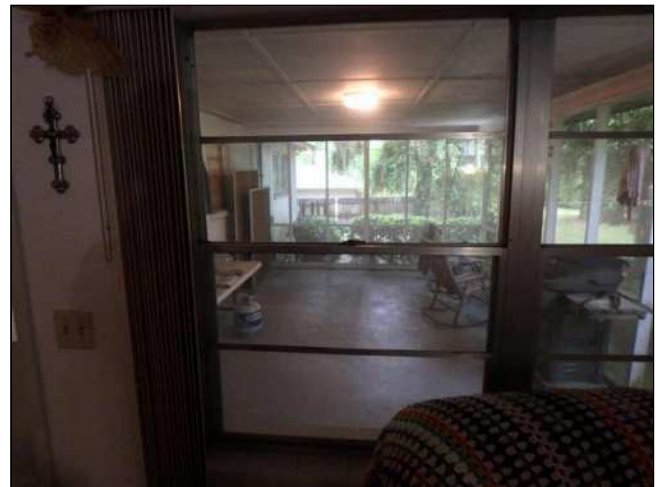
8.3 (5) LEFT SIDE FAMILY ROOM WINDOWS DO NOT REMAIN IN THE "UP" POSITION. Condition may be due to damaged / detached balancer springs.
