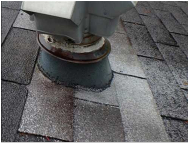
1.2(2) EXPOSED FLASHING (Picture 2)
