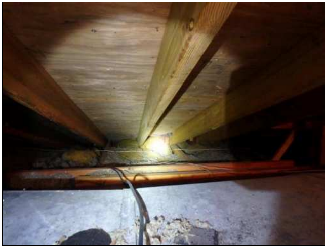
5.0(1) ROOF FRAMING (Picture 3)
