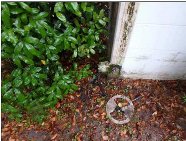
1.6(1) DOWNSPOUTS / ROOF DRAINS (Picture 1)
