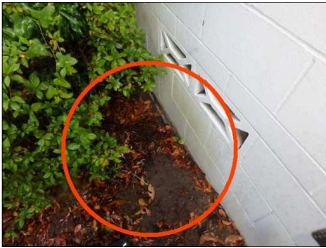
3.4(2) SITE GRADING (Picture 1)
