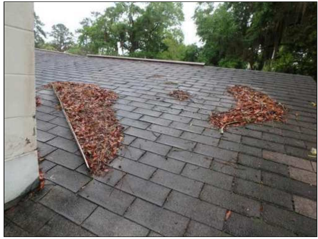
1.0(3) ROOF COVERING (Picture 2)
