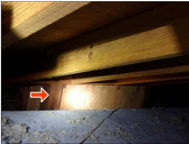
5.6 SKYLIGHT ENCLOSURE (Picture 3)
