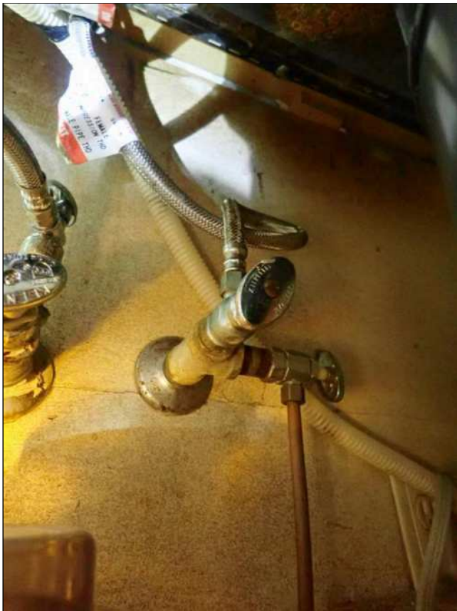
6.0(3) PLUMBING / SINK(S) (Picture 1)
