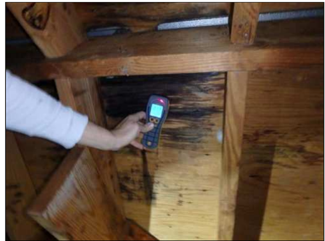
5.1(1) ROOF DECK / SHEATHING (Picture 2)
