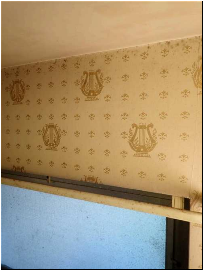
7.27(1) WALLS / CEILING (Picture 3)
