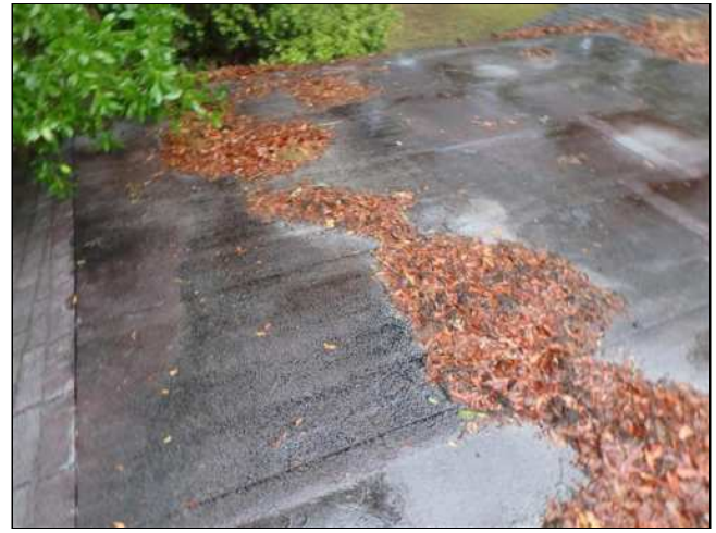
1.1(1) ROOF COVERING 2 (Picture 1)
