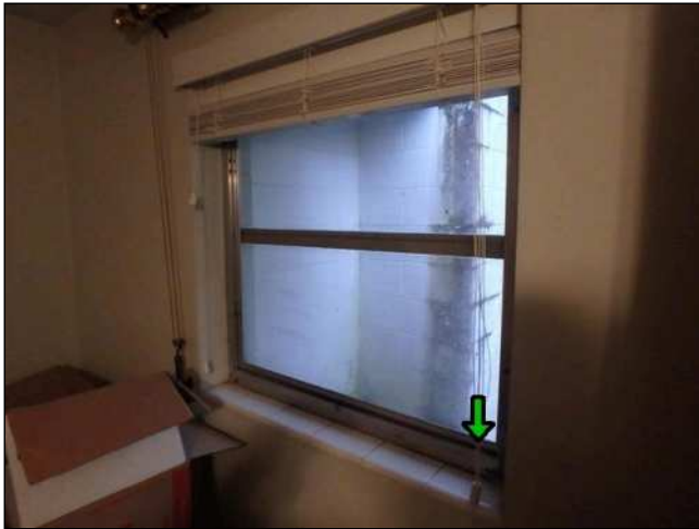
8.3 (4) MISSING CRANKS / HARDWARE OBSERVED AT REAR AND RIGHT SIDE WINDOWS OF RIGHT FRONT BEDROOM, THE REAR FAMILY ROOM WINDOWS AND THE FRONT WINDOWS AT LEFT FRONT BEDROOM. Condition may make window difficult to operate. Windows functioned normally at time of inspection.
