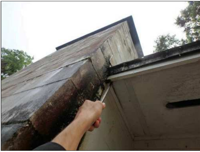
1.8(3) FASCIA / SOFFITS (Picture 5)
