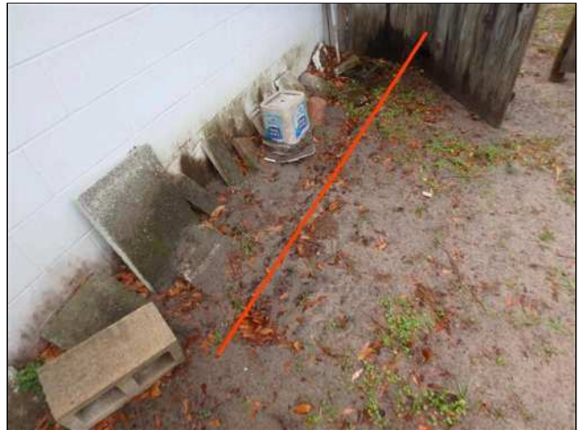
3.4(1) SITE GRADING (Picture 4)
