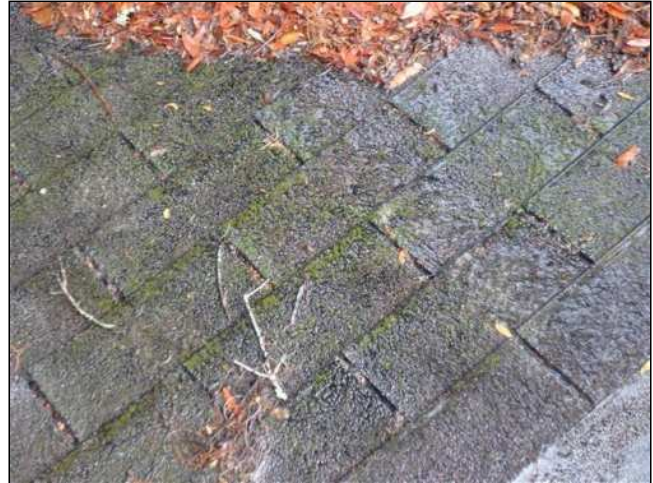
1.0(1) ROOF COVERING (Picture 2)
