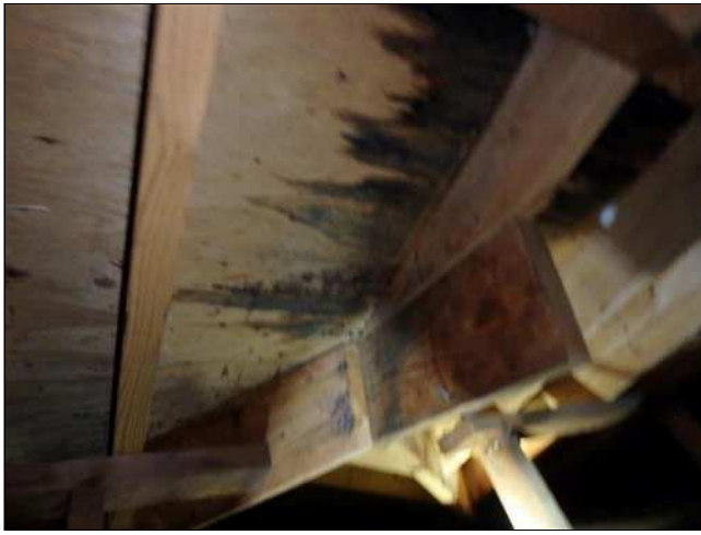
5.1(3) ROOF DECK / SHEATHING (Picture 1)
