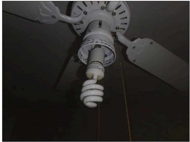
8.6(1) CEILING FANS (Picture 2)
