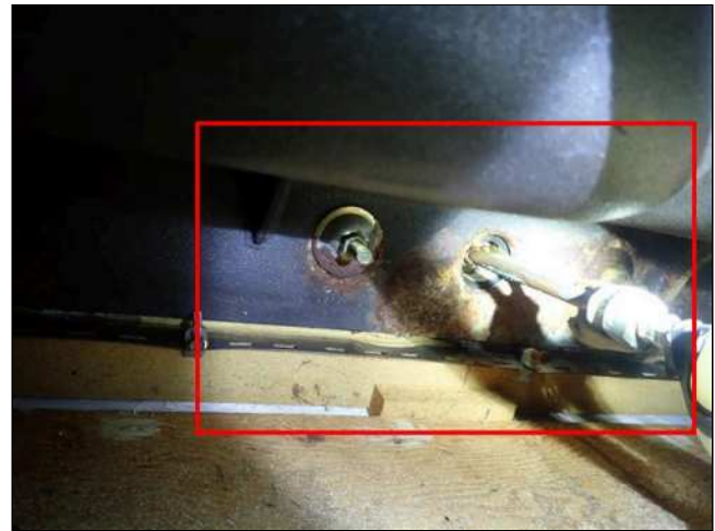
6.0(1) PLUMBING / SINK(S) (Picture 2)
