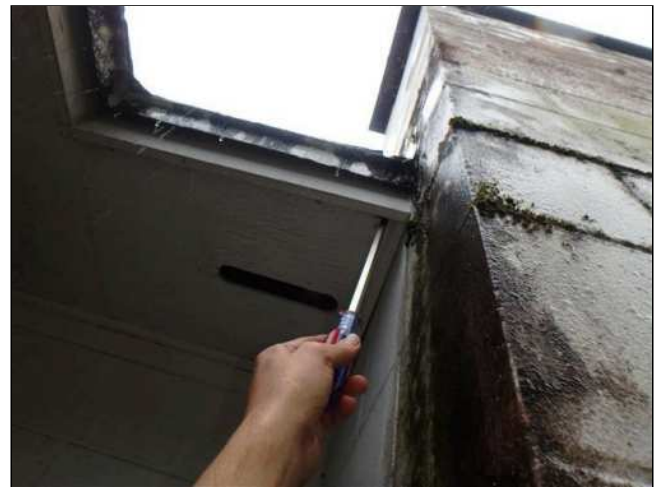
1.8(3) FASCIA / SOFFITS (Picture 4)
