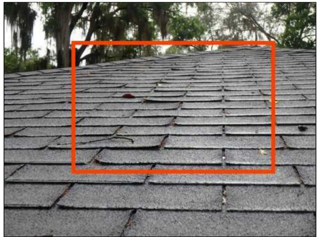
1.0(6) ROOF COVERING (Picture 5)
