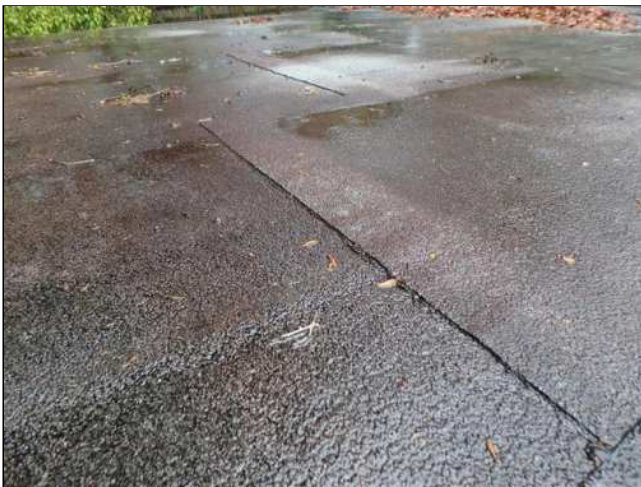
1.1(3) ROOF COVERING 2 (Picture 1)
