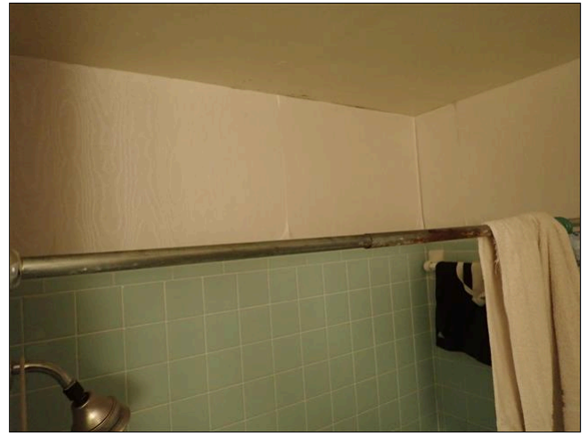
7.7 WALLS / CEILING (Picture 1)
