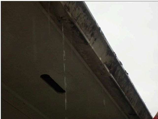
1.7(4) RAIN GUTTERS / EAVESTROUGHES (Picture 4)
