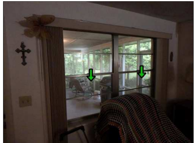
8.3(5) INTERIOR WINDOWS (Picture 1)
