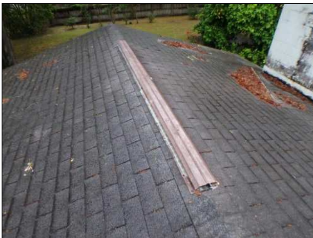
1.2 (4) LACK OF KICK-OUT FLASHING OBSERVED AT THE EXTERIOR SIDING (CHIMNEY) / ROOF LINE INTERFACE. Condition may allow roof drainage / rainwater to drain onto underlying materials, which may lead to moisture related damage. Condition of latent materials was not visible & could not be fully inspected. Hidden damage may exist.
