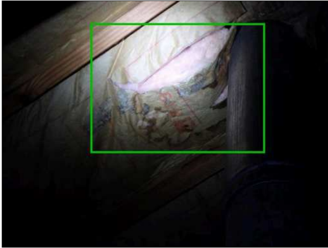
4.4(1) WALLS / CEILINGS (Picture 1)
