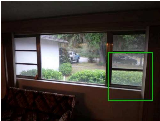
8.3(7) INTERIOR WINDOWS (Picture 1)
