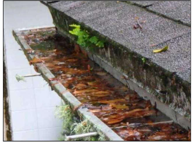
1.7 (2) STAINING OBSERVED AT DOWNSPOUT AND/OR GUTTER SYSTEM SEAMS. THIS IS USUALLY AN INDICATION OF SEAM LEAKS. Full gutters and/or downspout blockage is the primary cause of leaks at the seams of gutters / downspouts. Annual / Bi-annual maintenance may be required in order to ensure gutter / downspout integrity. Pictures shown are a representative number of affected areas.
