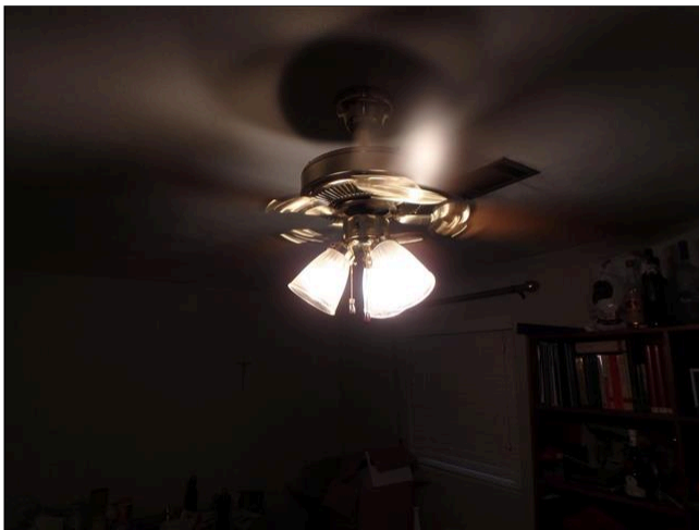
8.6(2) CEILING FANS (Picture 1)
