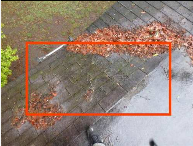
1.0(1) ROOF COVERING (Picture 1)
