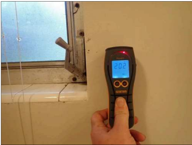
7.18 WALLS / CEILING (Picture 6)
