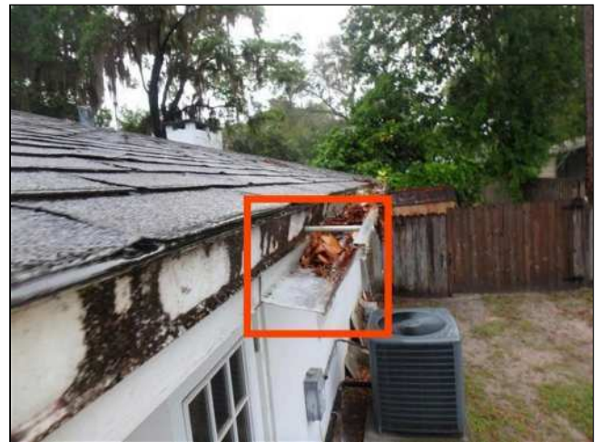
1.7 (4) FRONT GUTTER SYSTEM IS LEAKING / HAS FAILED & HAS HOLES DRILLED INTO THE BOTTOM OF THE GUTTER SYSTEM. Current condition may be due to leaves / debris accumulation in the gutter system & related downspouts. RECOMMEND HAVING A LICENSED HANDYMAN OR CONTRACTOR EVALUATE / REMEDY AS NEEDED.
