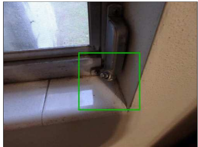
8.3(4) INTERIOR WINDOWS (Picture 2)
