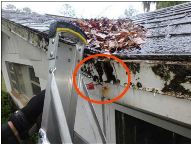
1.8(3) FASCIA / SOFFITS (Picture 1)
