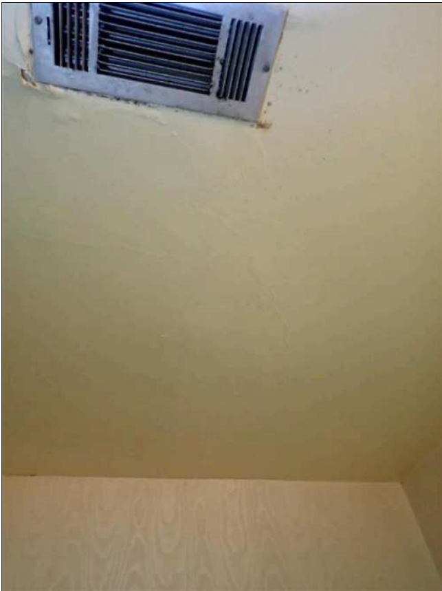
7.7 WALLS / CEILING (Picture 16)
