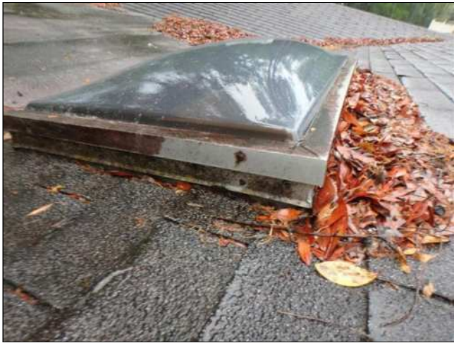
1.2(5) EXPOSED FLASHING (Picture 1)
