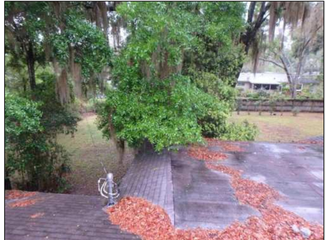
1.0(2) ROOF COVERING (Picture 2)
