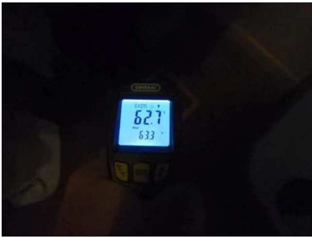
12.1(1) COOLING SYSTEM (Picture 1)
