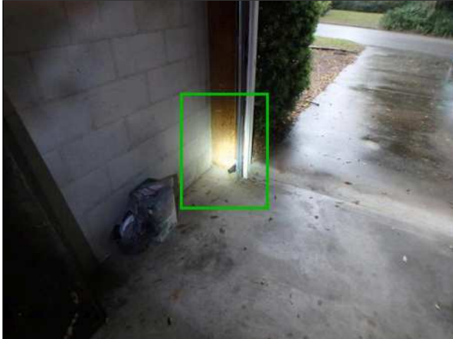
4.4(2) WALLS / CEILINGS (Picture 1)
