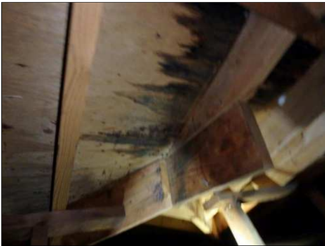
5.1(1) ROOF DECK / SHEATHING (Picture 1)
