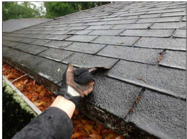
1.0(6) ROOF COVERING (Picture 1)
