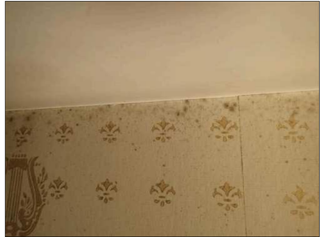
7.27(1) WALLS / CEILING (Picture 4)
