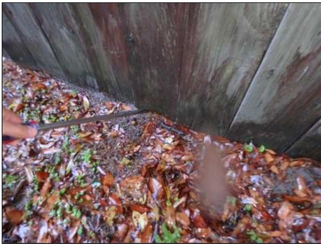
3.2 (2) WOOD DECAY AND/OR DAMAGE OBSERVED AT FENCING MATERIALS. Wood decay / damage may deteriorate the integrity / rigidity of affected materials over time.
