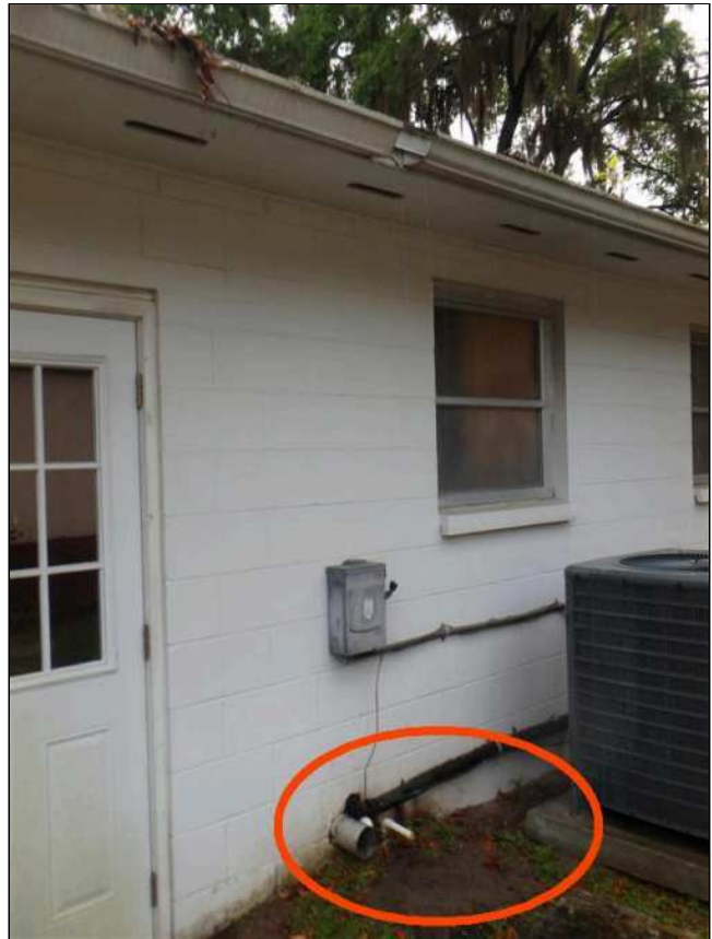
3.4(1) SITE GRADING (Picture 2)
