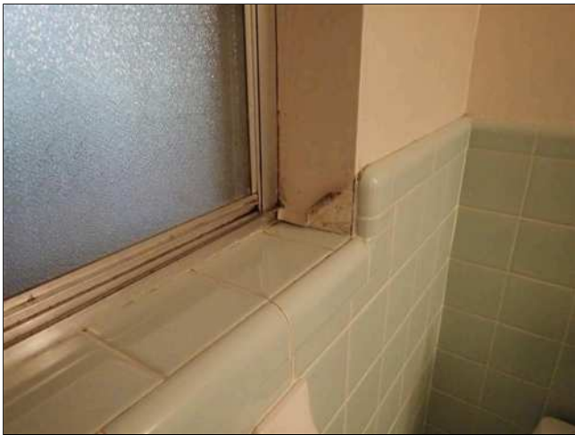
7.7 WALLS / CEILING (Picture 14)
