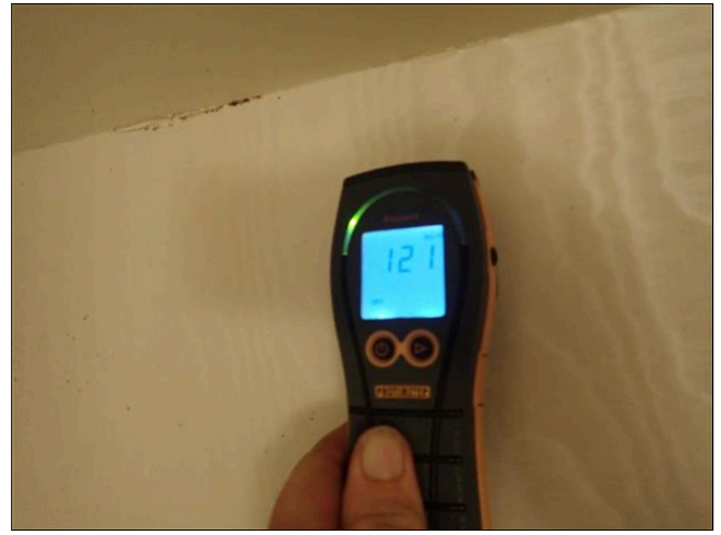
7.7 WALLS / CEILING (Picture 13)
