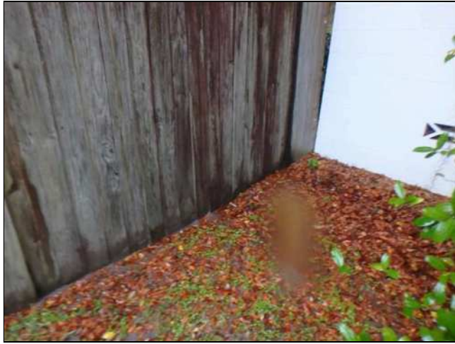
3.2 (2) WOOD DECAY AND/OR DAMAGE OBSERVED AT FENCING MATERIALS. Wood decay / damage may deteriorate the integrity / rigidity of affected materials over time.
