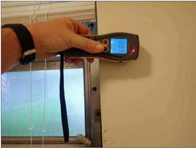
7.18 WALLS / CEILING (Picture 4)
