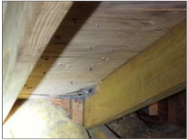
5.0(1) ROOF FRAMING (Picture 4)
