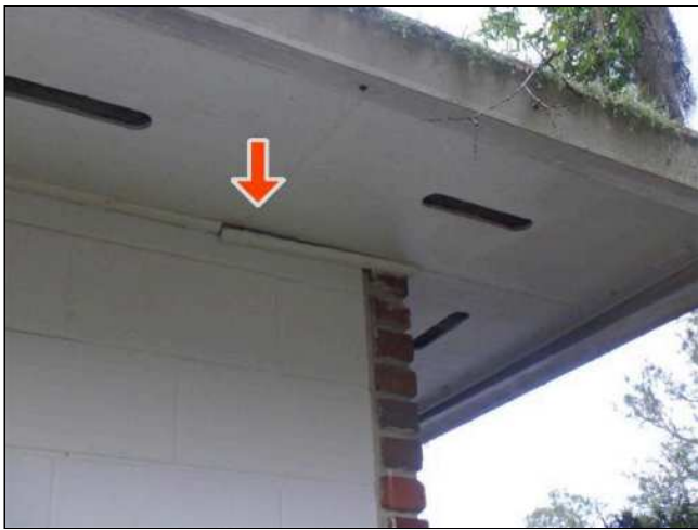
1.8(2) FASCIA / SOFFITS (Picture 3)
