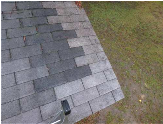
1.0(4) ROOF COVERING (Picture 1)
