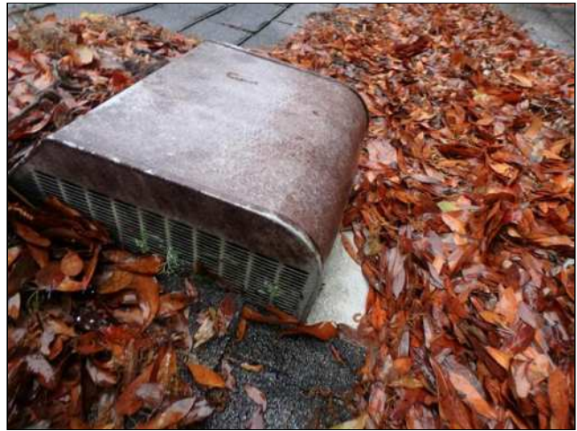
1.2(5) EXPOSED FLASHING (Picture 2)
