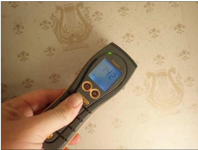
7.27(2) WALLS / CEILING (Picture 9)
