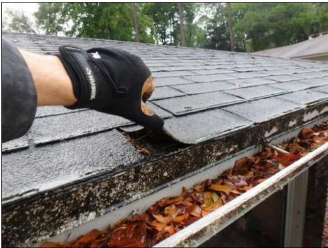
1.0(6) ROOF COVERING (Picture 4)
