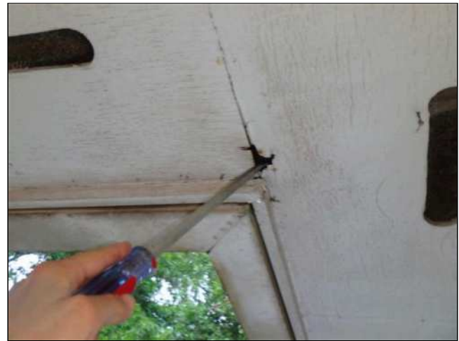
1.8(3) FASCIA / SOFFITS (Picture 2)
