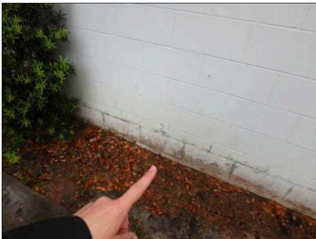
9.0(1) FOUNDATION WALLS (Picture 1)
