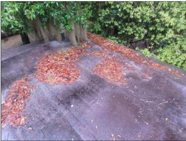
1.1(1) ROOF COVERING 2 (Picture 2)
