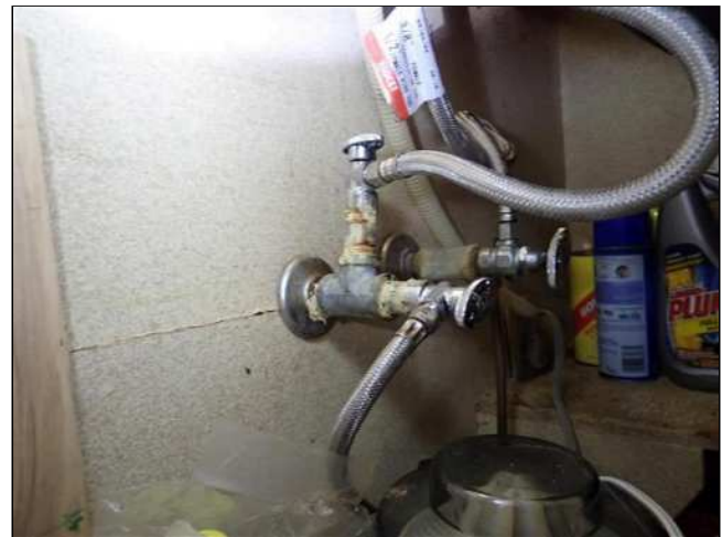
6.0(3) PLUMBING / SINK(S) (Picture 2)
