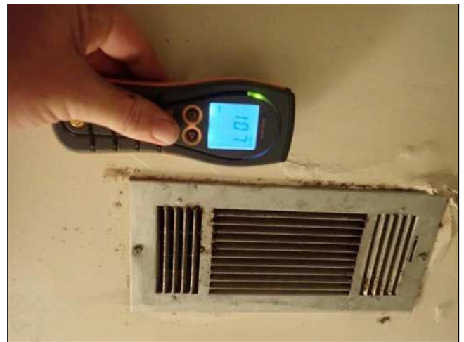
7.7 WALLS / CEILING (Picture 11)
