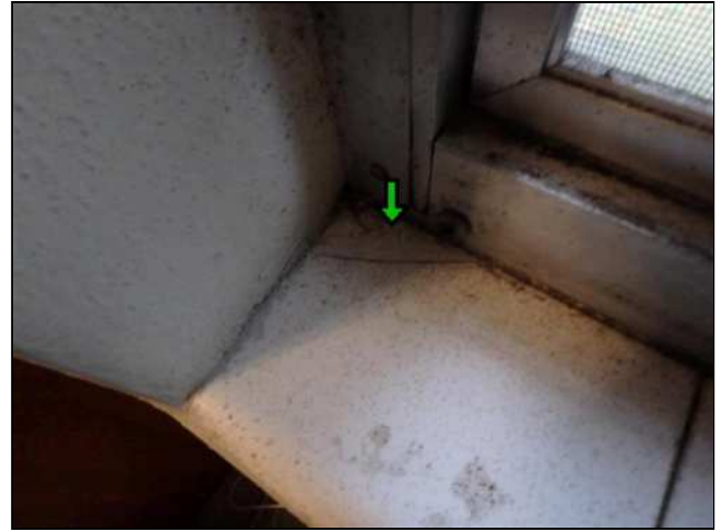
8.3 (4) MISSING CRANKS / HARDWARE OBSERVED AT REAR AND RIGHT SIDE WINDOWS OF RIGHT FRONT BEDROOM, THE REAR FAMILY ROOM WINDOWS AND THE FRONT WINDOWS AT LEFT FRONT BEDROOM. Condition may make window difficult to operate. Windows functioned normally at time of inspection.
