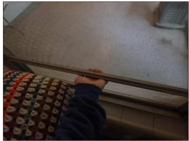
8.3(5) INTERIOR WINDOWS (Picture 5)
