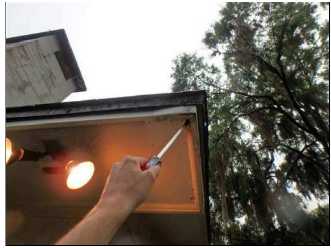
1.8(3) FASCIA / SOFFITS (Picture 6)
