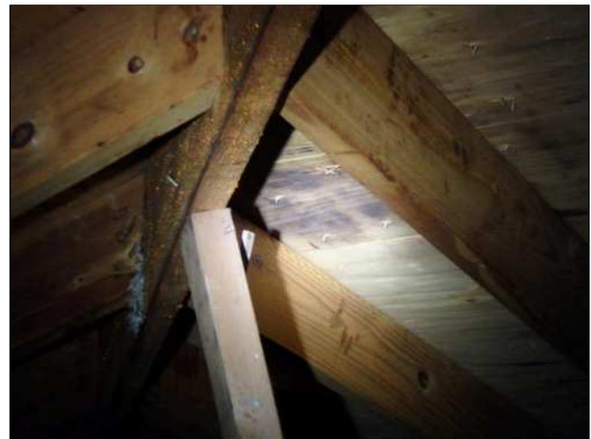
5.1(2) ROOF DECK / SHEATHING (Picture 2)
