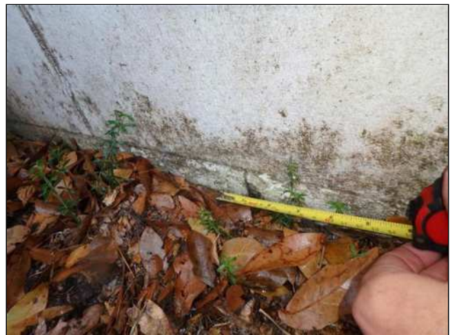
9.0(1) FOUNDATION WALLS (Picture 2)
