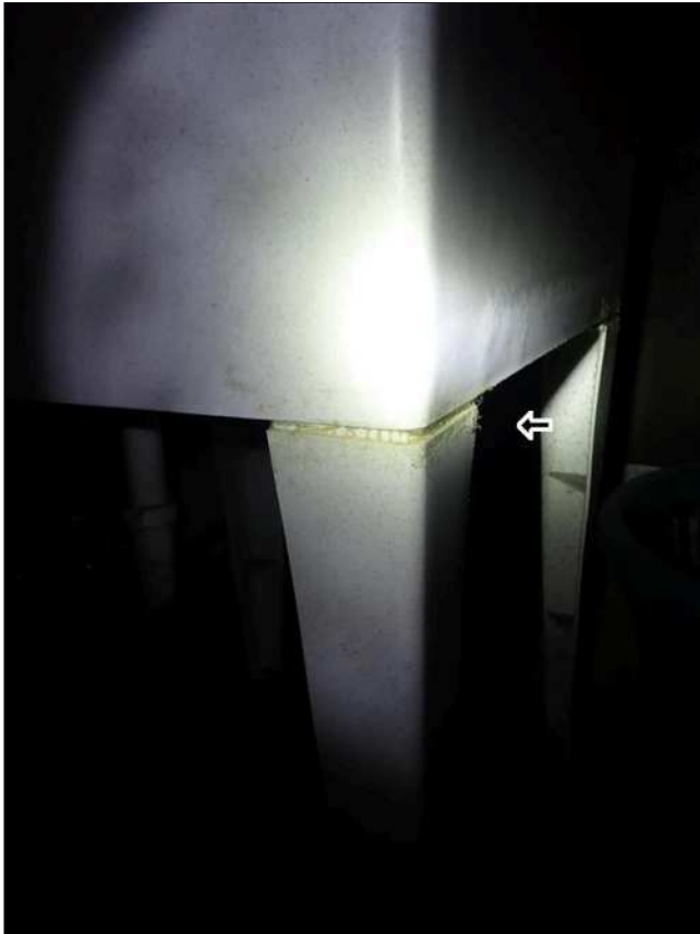
14.5(2) LAUNDRY SINK (Picture 3)
