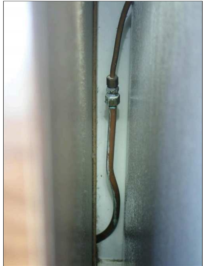
6.0(4) PLUMBING / SINK(S) (Picture 2)
