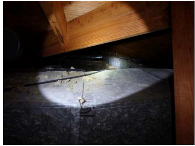
5.0(4) ROOF FRAMING (Picture 2)
