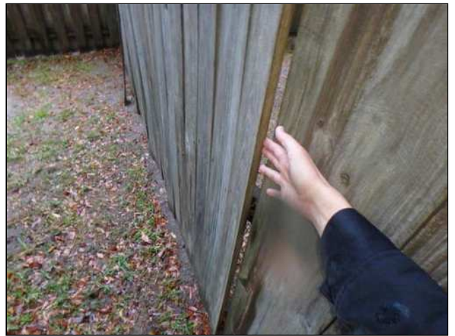
3.2 (2) WOOD DECAY AND/OR DAMAGE OBSERVED AT FENCING MATERIALS. Wood decay / damage may deteriorate the integrity / rigidity of affected materials over time.
