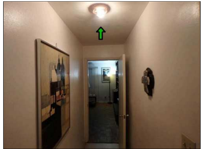
8.7(2) ELECTRIC / DEVICES (Picture 1)
