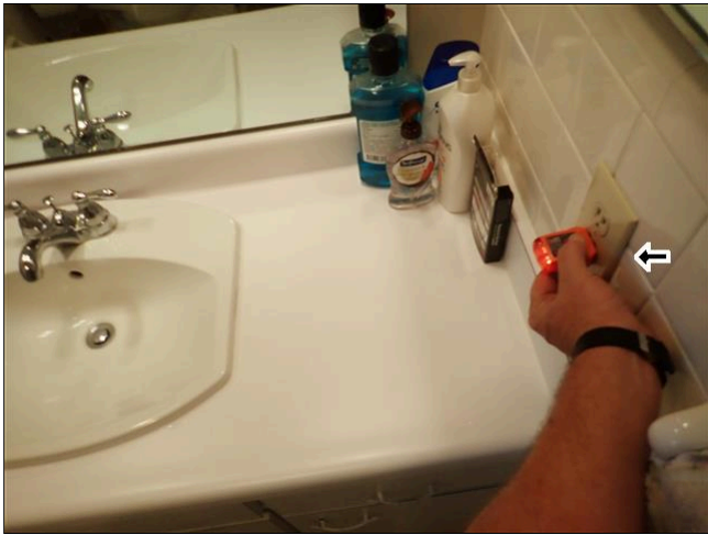
7.20 ELECTRIC / GFCI (Picture 1)
