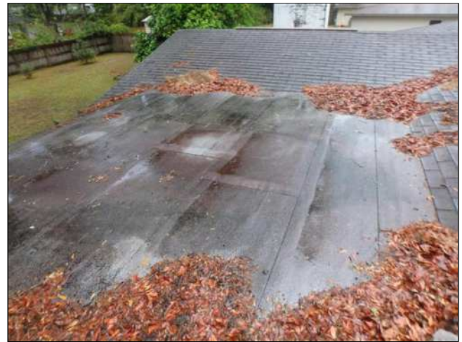
1.1(2) ROOF COVERING 2 (Picture 1)
