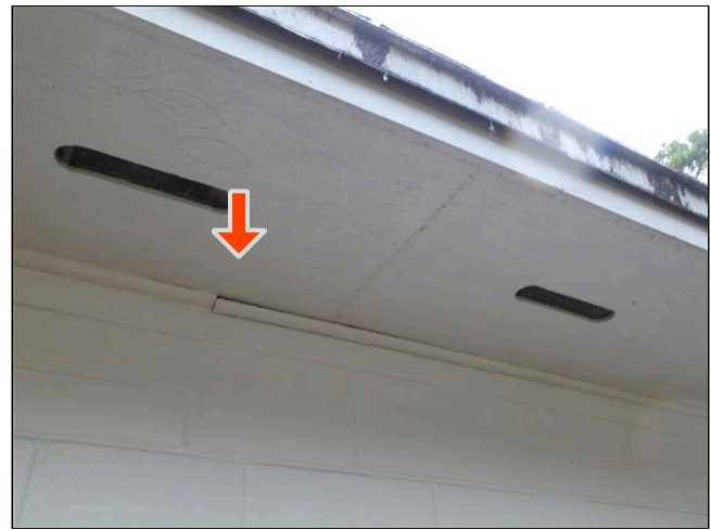
1.8(2) FASCIA / SOFFITS (Picture 4)
