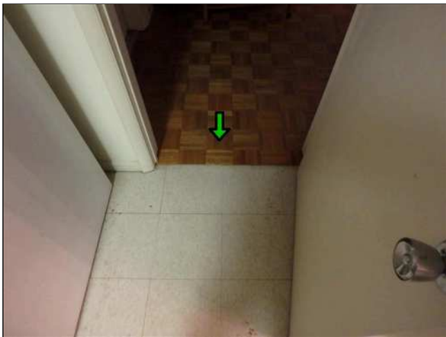
8.2(1) FLOORS (SLAB) (Picture 1)
