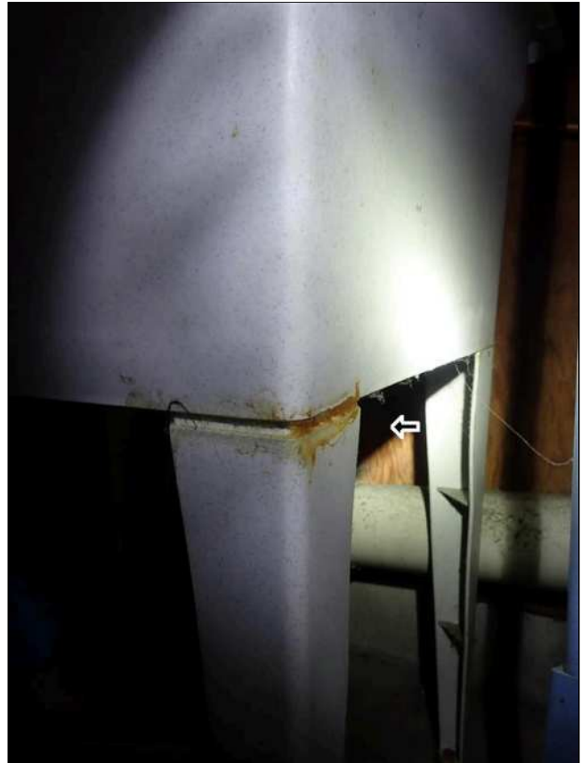
14.5(2) LAUNDRY SINK (Picture 4)
