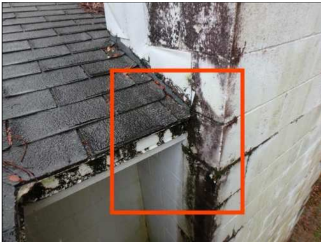
1.2(4) EXPOSED FLASHING (Picture 2)
