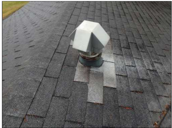
1.0(4) ROOF COVERING (Picture 2)
