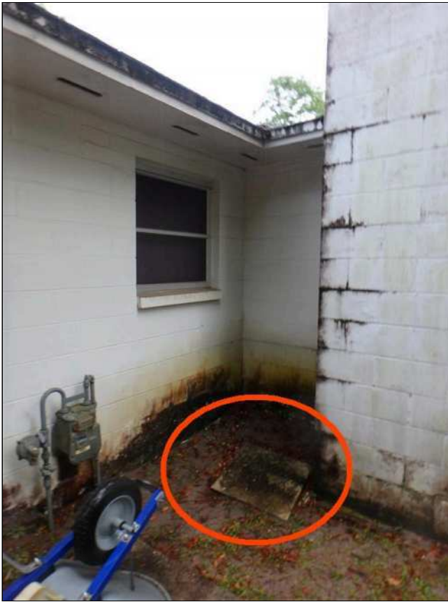
3.4(1) SITE GRADING (Picture 5)
