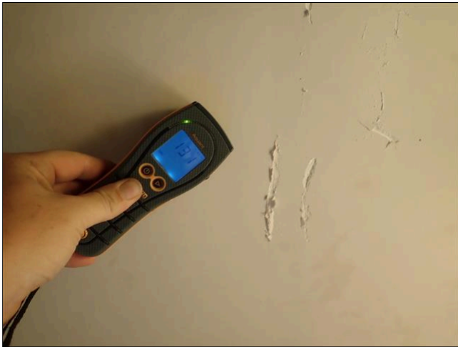
7.27(2) WALLS / CEILING (Picture 7)
