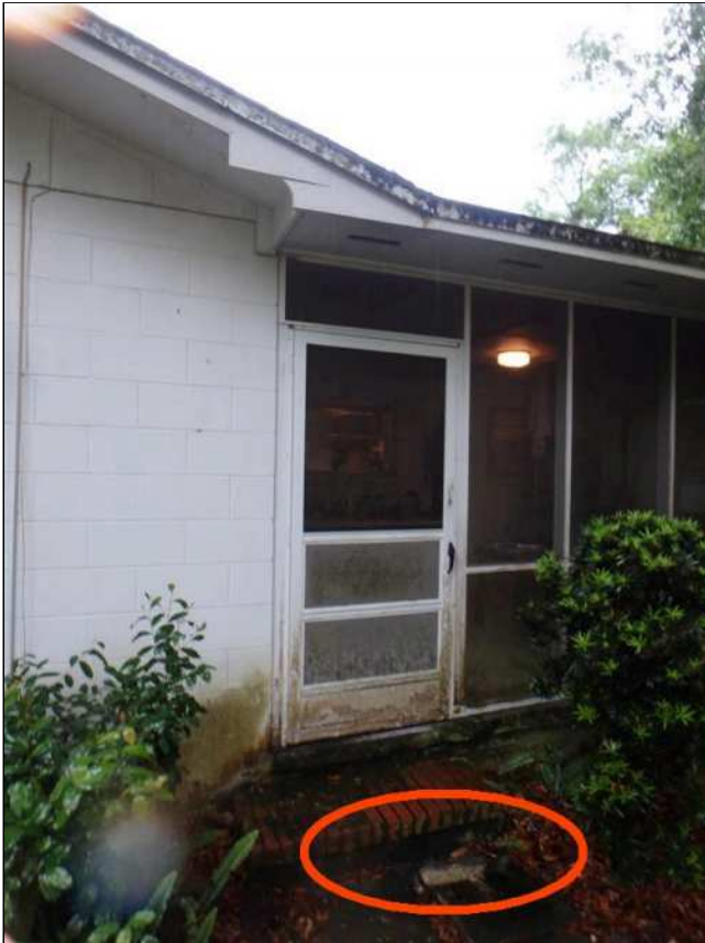
3.4(1) SITE GRADING (Picture 7)
