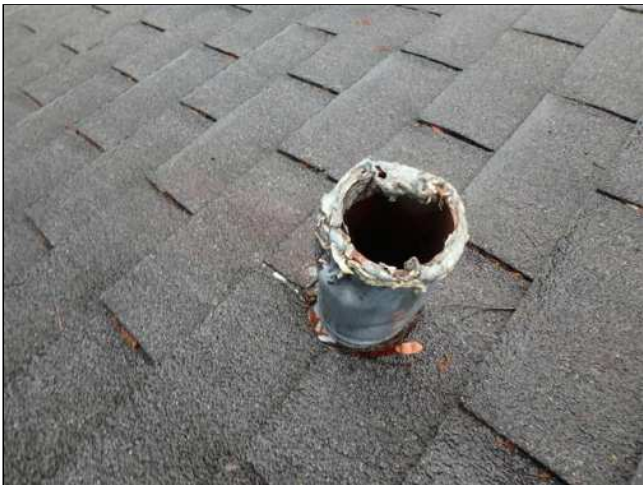
1.2(1) EXPOSED FLASHING (Picture 3)
