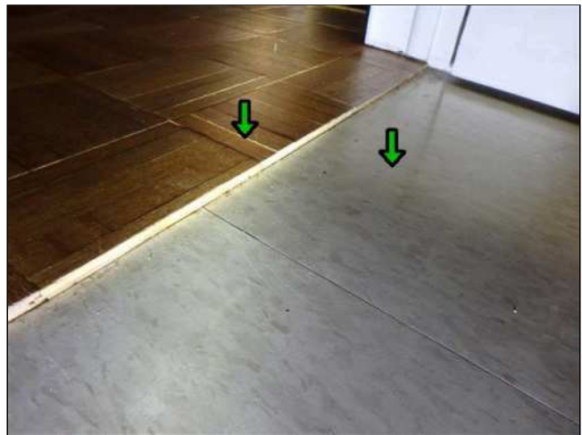
8.2(1) FLOORS (SLAB) (Picture 2)
