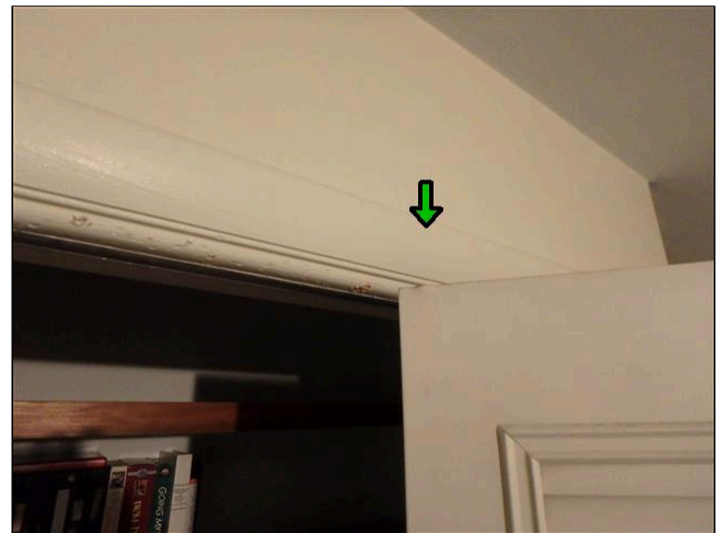
8.5(2) INTERIOR CLOSET DOOR(S) (Picture 4)
