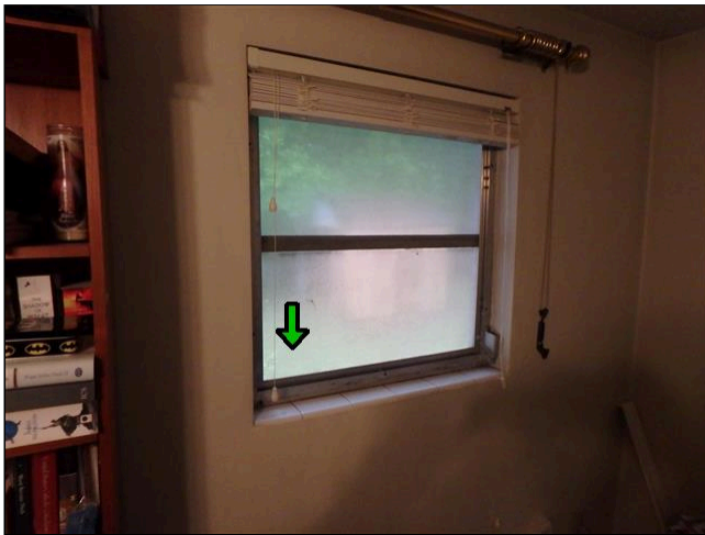
8.3(3) INTERIOR WINDOWS (Picture 1)
