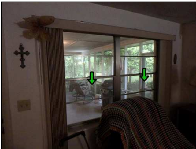
8.3 (5) LEFT SIDE FAMILY ROOM WINDOWS DO NOT REMAIN IN THE "UP" POSITION. Condition may be due to damaged / detached balancer springs.
