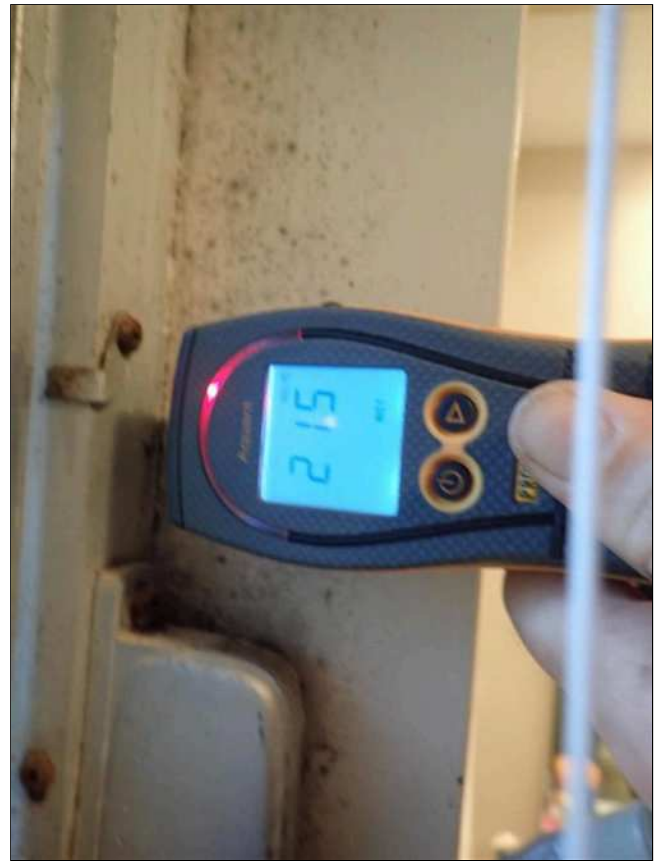
7.18 WALLS / CEILING (Picture 3)
