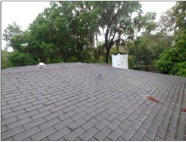
1.0(7) ROOF COVERING (Picture 2)
