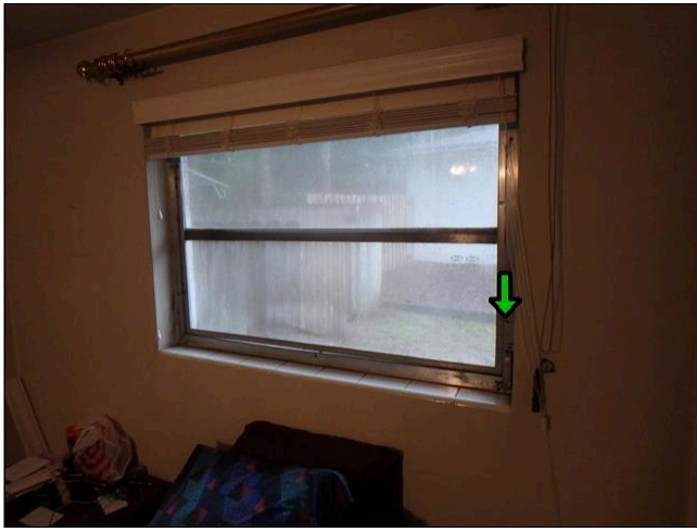
8.3(4) INTERIOR WINDOWS (Picture 3)
