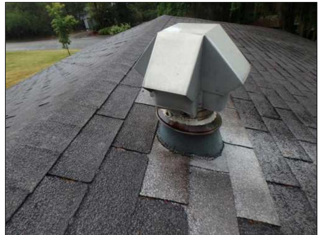
1.2(2) EXPOSED FLASHING (Picture 1)
