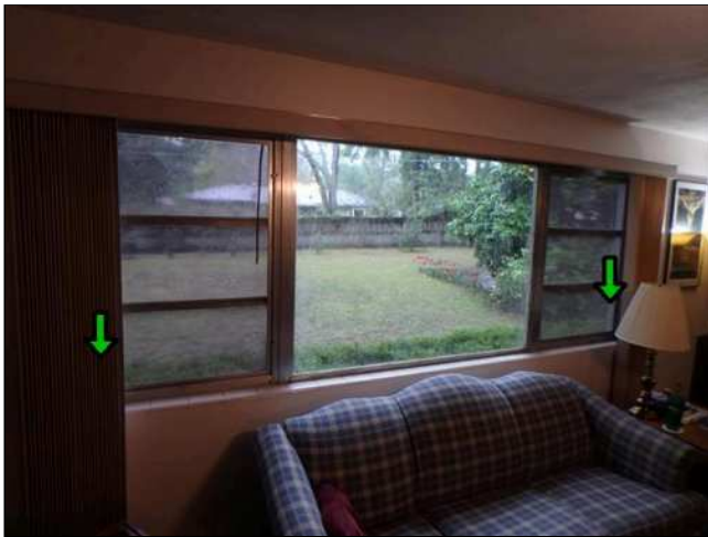
8.3(4) INTERIOR WINDOWS (Picture 5)
