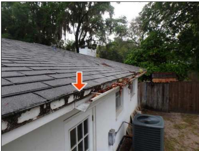
1.7 (4) FRONT GUTTER SYSTEM IS LEAKING / HAS FAILED & HAS HOLES DRILLED INTO THE BOTTOM OF THE GUTTER SYSTEM. Current condition may be due to leaves / debris accumulation in the gutter system & related downspouts. RECOMMEND HAVING A LICENSED HANDYMAN OR CONTRACTOR EVALUATE / REMEDY AS NEEDED.
