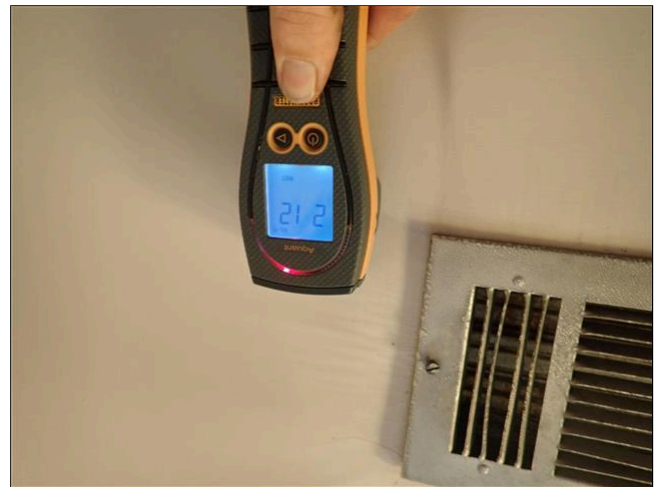
7.27(2) WALLS / CEILING (Picture 6)
