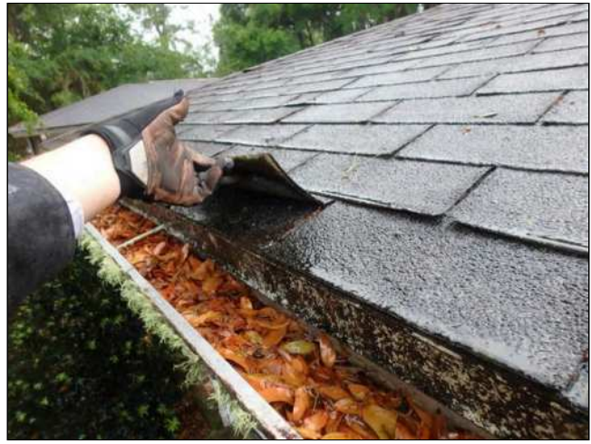
1.0(6) ROOF COVERING (Picture 3)
