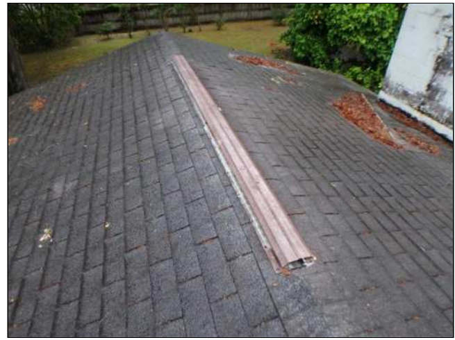
1.2(3) EXPOSED FLASHING (Picture 1)
