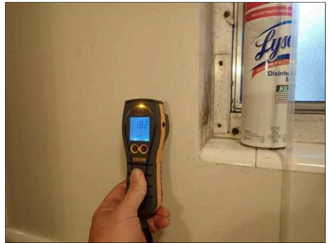
7.18 WALLS / CEILING (Picture 7)
