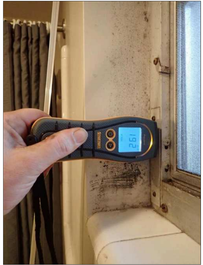
7.18 WALLS / CEILING (Picture 9)
