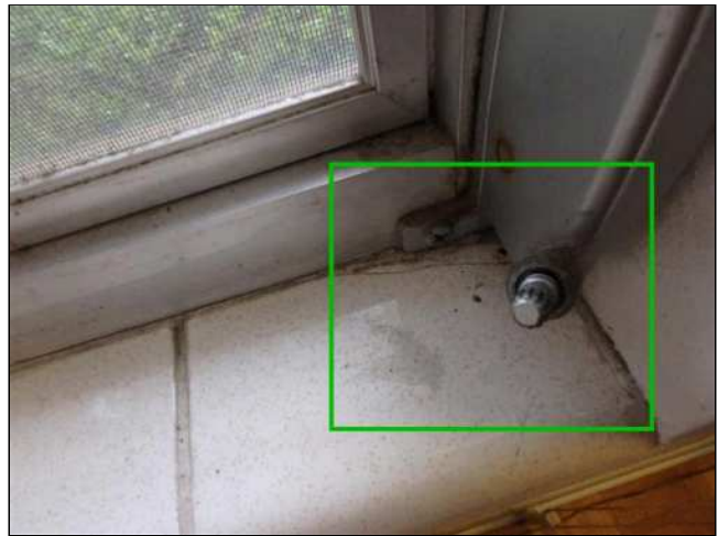
8.3(4) INTERIOR WINDOWS (Picture 6)
