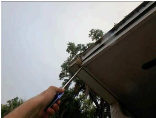
1.8(3) FASCIA / SOFFITS (Picture 3)
