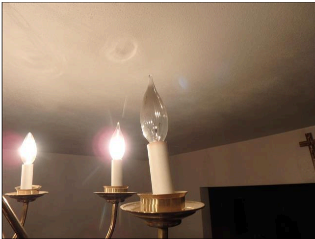
8.7(1) ELECTRIC / DEVICES (Picture 2)
