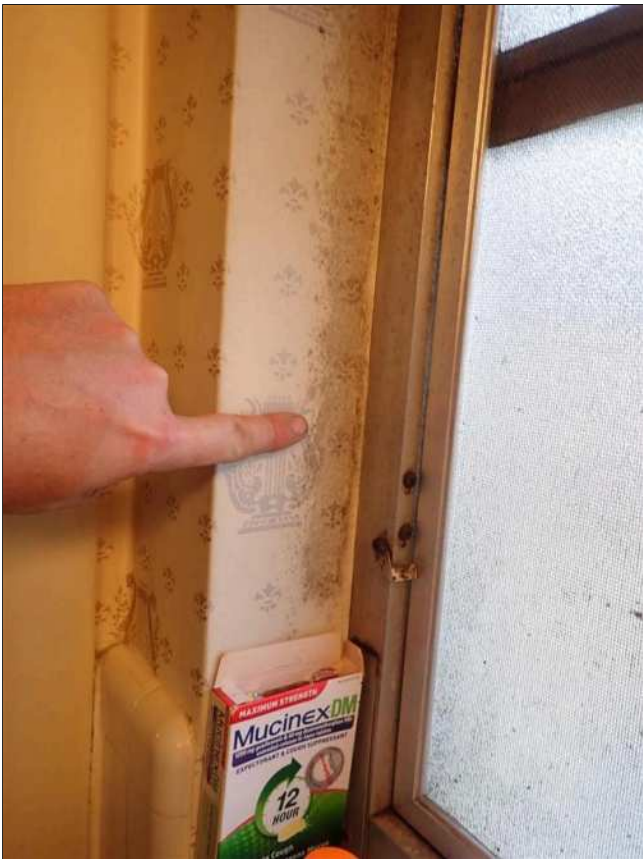
7.27(1) WALLS / CEILING (Picture 1)
