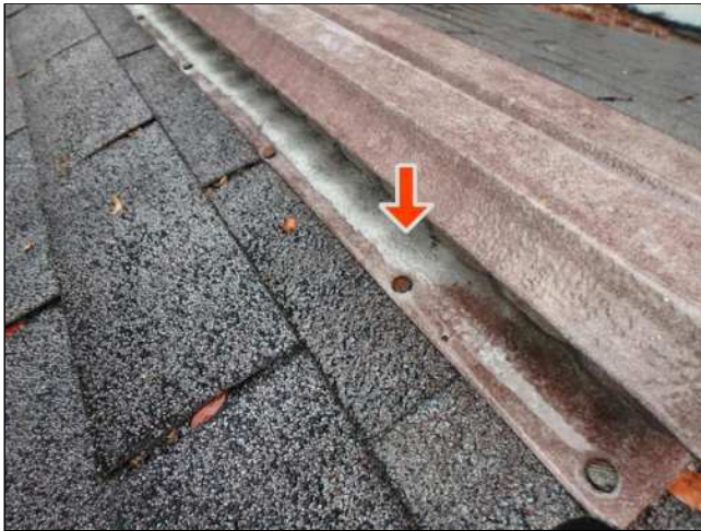
1.2(3) EXPOSED FLASHING (Picture 2)
