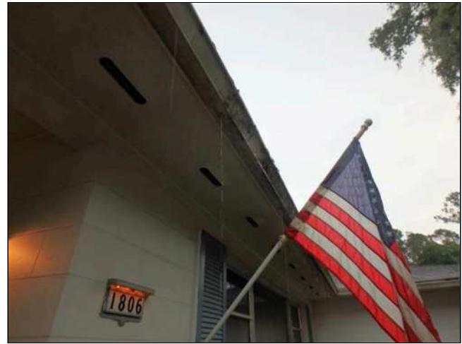
1.7(4) RAIN GUTTERS / EAVESTROUGHES (Picture 3)
