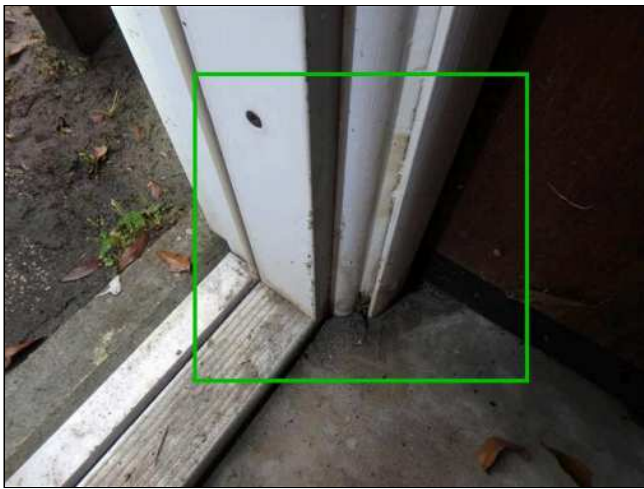
4.4(3) WALLS / CEILINGS (Picture 1)
