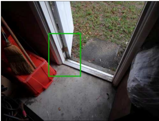
4.9 ENTRY DOOR(S) (Picture 1)
