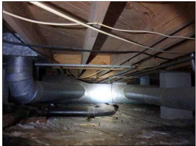
9.6 CRAWLSPACE ENTRY / ACCESS (Picture 1)
