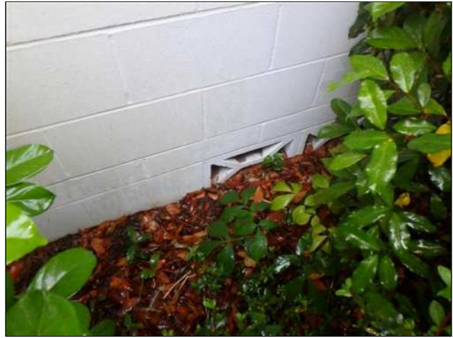
9.5 CRAWLSPACE VENTILATION PROVISIONS (Picture 1)
