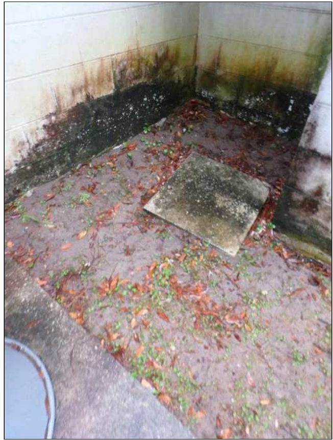
3.4(1) SITE GRADING (Picture 6)
